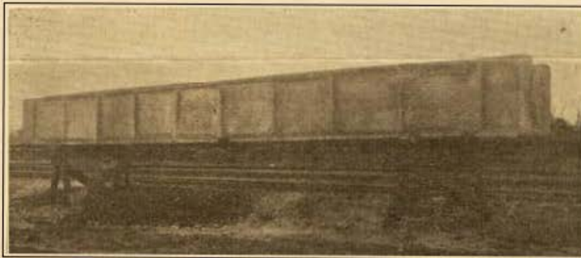
FIG. 1.—LEASIDE GIRDBERS PRIOR TO APPLICATION OF GUNITE
