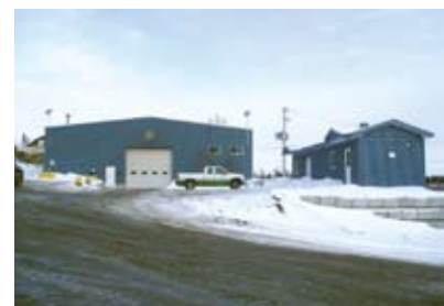
Fig. 14: Concrete plant (at left) and concrete laboratory (at right)
