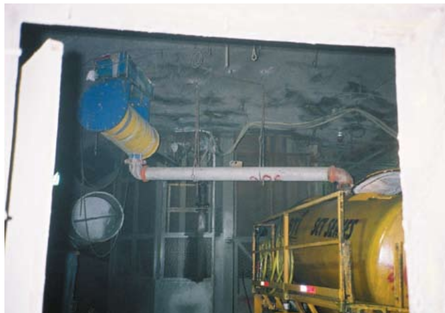
Fig. 6: Loading self-consolidating shotcrete into the transmixer
