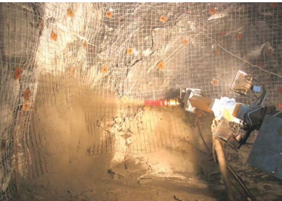
Fig. 8: Application of shotcrete in one stope
