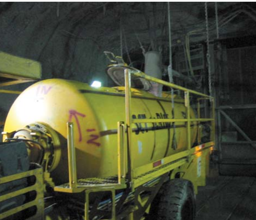
Fig. 4: Old system of receiving concrete
