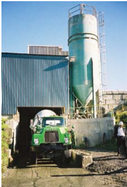
Fig. 7: Concrete plant in use by Beton Fournier at Cadillac
