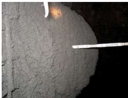
Fig. 9: Thickness of fresh shotcrete on the wall
