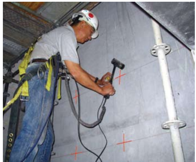
Impulse-response testing on the inside surface of the panel
