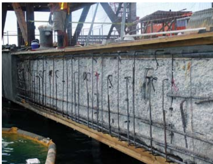
Prepared surface with timber side shutters
