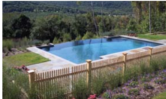
A westerly view of the pool area shows the drastic slope of the building site. In the shadows of the edge wall is a foot ledge that continues the length of the pool
