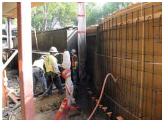
Two means of material placement were used on this job. Concrete pumping (above) was used in some elements by taking the nozzle off at areas to be vibrated. The pump-and-shoot approach (below) was used on most of the vertical work
