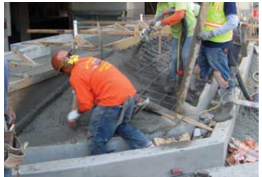
Two means of material placement were used on this job. Concrete pumping (above) was used in some elements by taking the nozzle off at areas to be vibrated. The pump-and-shoot approach (below) was used on most of the vertical work
