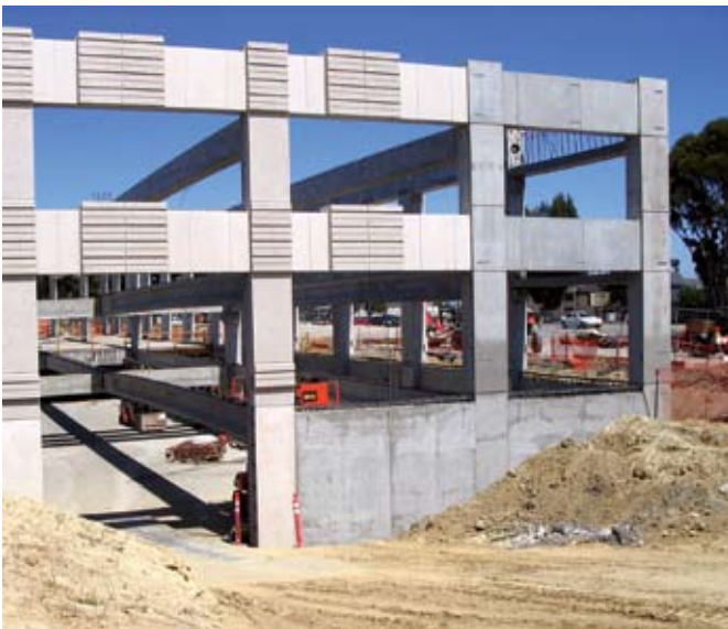
Completed basement-level shotcrete walls ready for waterproofing and structural backfill
