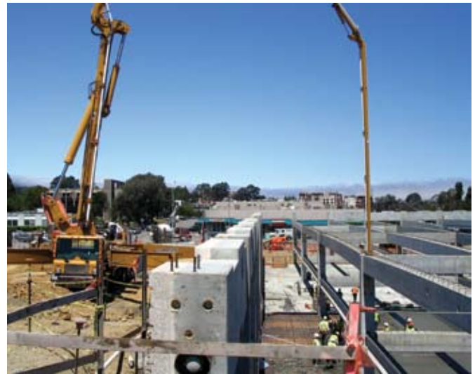
Placing the second floor deck
