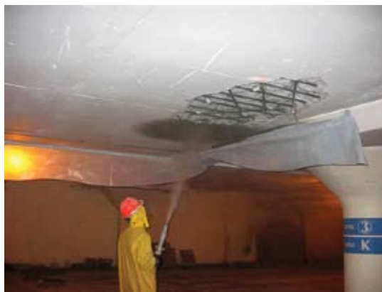
Dry-process shotcrete during placement overhead
