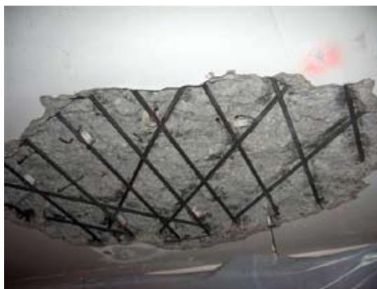
Prepared repair area with galvanic anodes
