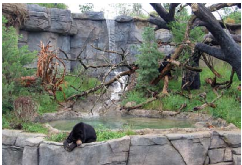
Shotcrete and hand-sculpted rock formations among habitat elements in Sun Bear exhibit
