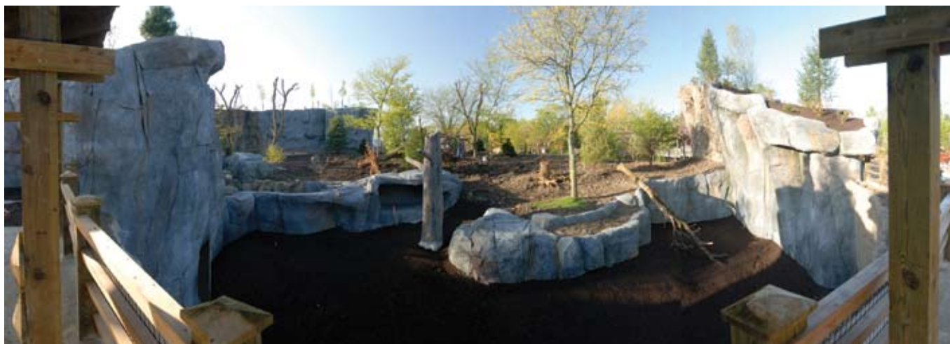
Shotcrete and hand-sculpted rock formations among habitat elements in the Markhor Exhibit
