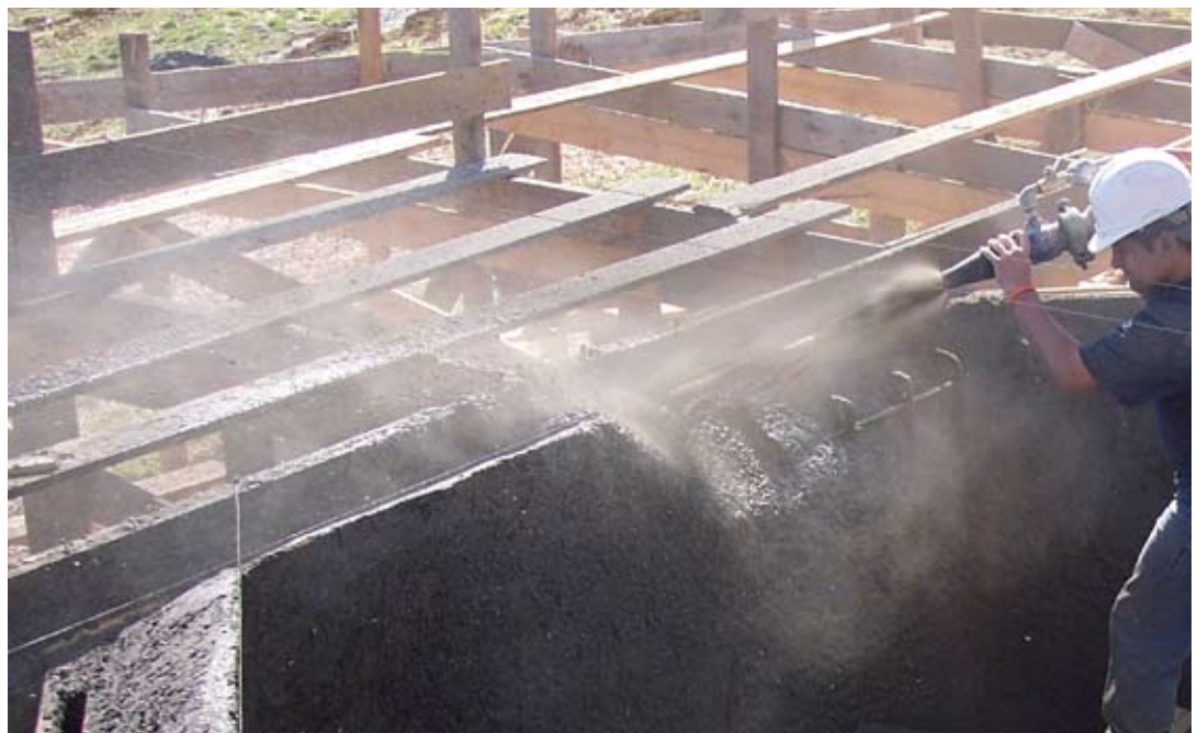
Shooting for exact tolerances on walls and edges creates ease of movement for water in transit. Shooting in tight tolerances also reduces preparation for the installation of the finish material (tile)
