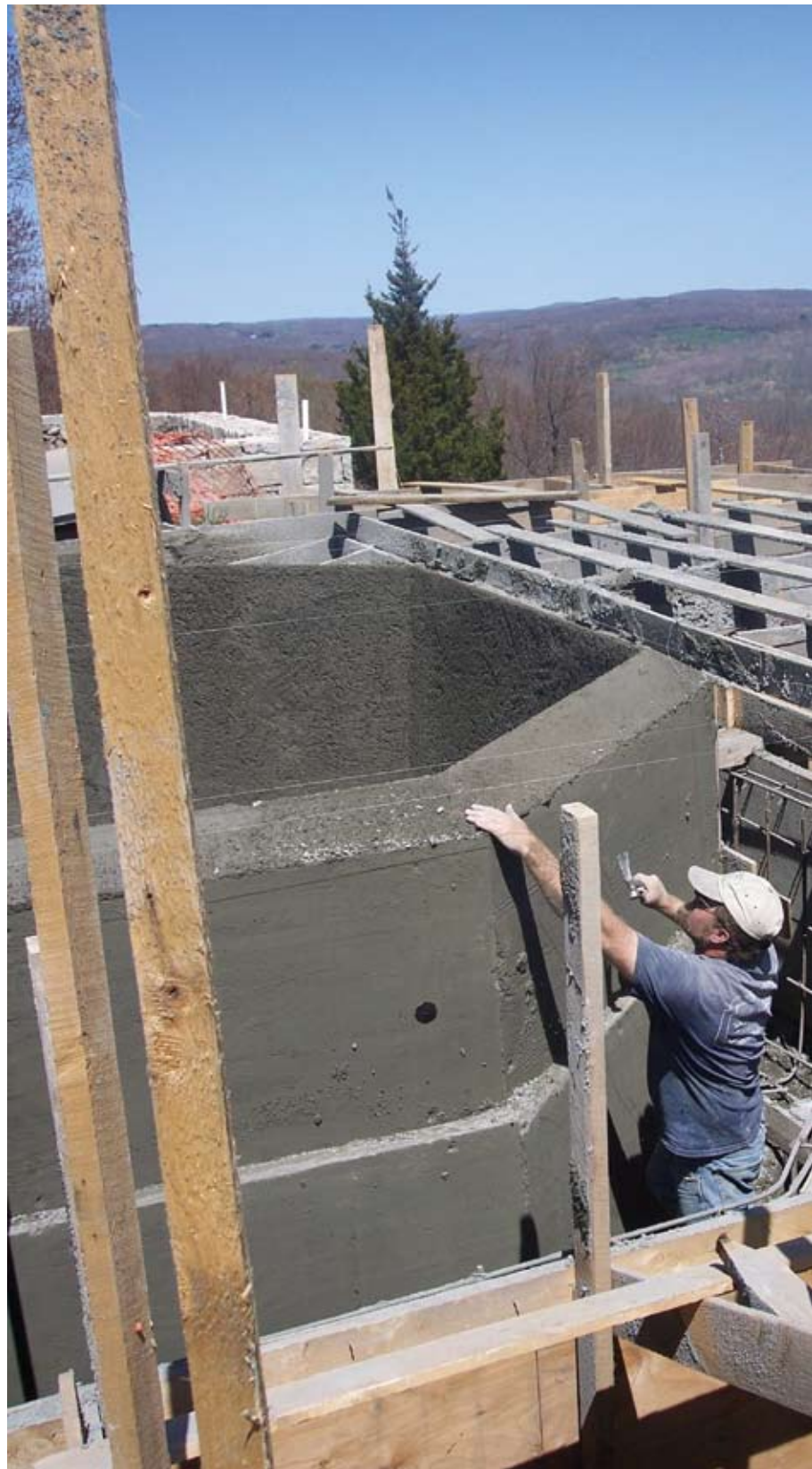
This picture depicts the denseness of the concrete. Thickness, tolerance, and uniformity of the shotcrete are shown, as well as the encapsulation of the reinforcement bar
