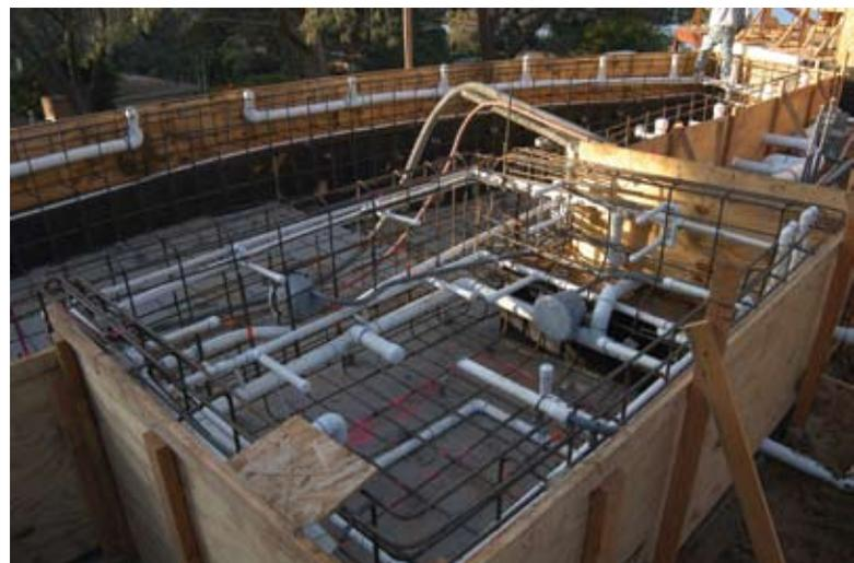
*The steel and plumbing for the pool, spa, and perimeter are completed after the upper pool forms are installed*
