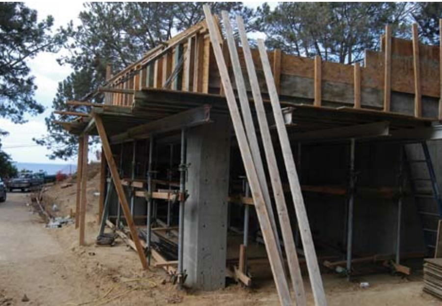
*The structural box that will support the pool and spa is installed. The top of the box is approximately 2 in. (50 mm) lower than the top of the pool finish elevation*
