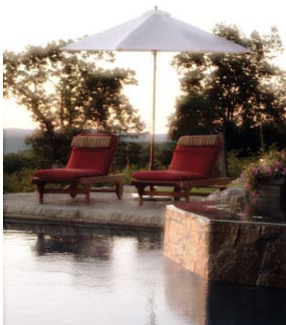
A medium gray plaster finish was used over the shotcrete structure to give it a reflective, inviting quality
