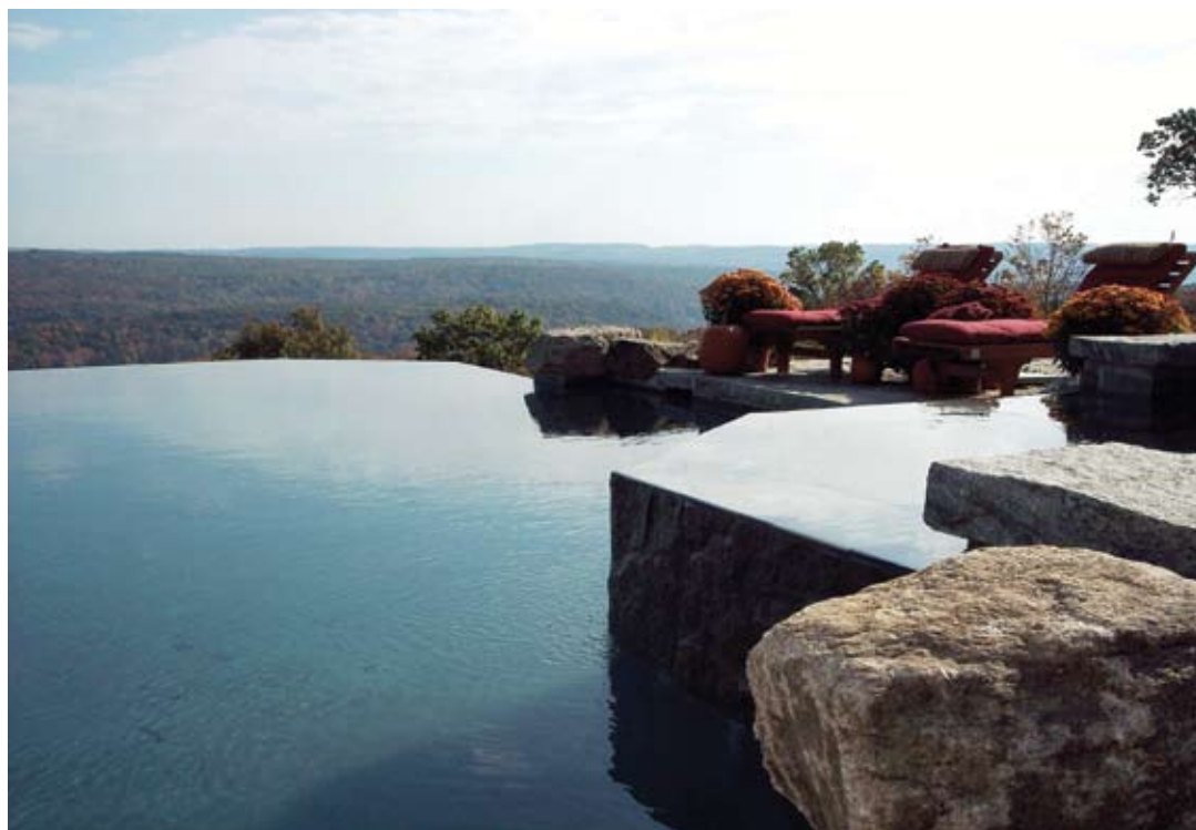
The spa wall design with its perimeter overflow was used to keep one's line-of-sight open. The water in transit over the edge mimics a sheet of glass and creates an illusion at the surface
