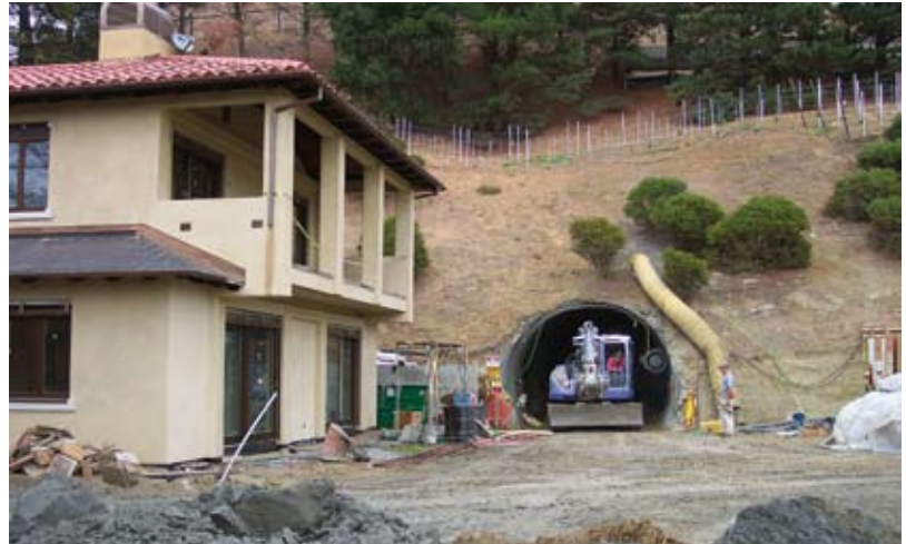
Fig. 1: Wine cave portal near owner's residence
