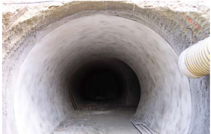
Fig. 2: Wine cave after application of spray-on waterproofing membrane
