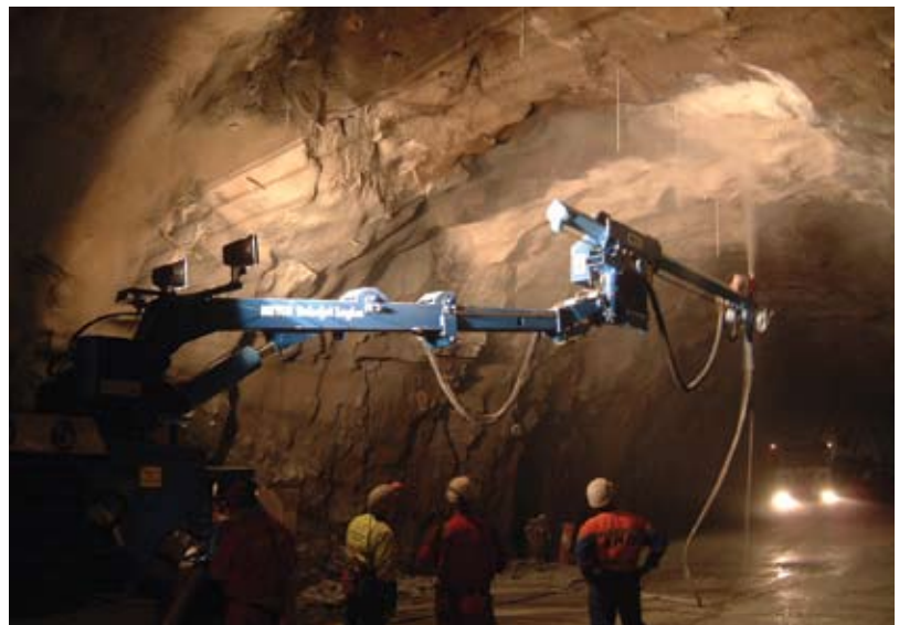
Fig. 3: Application at intersection with robotic sprayer, Nordoy Tunnel
