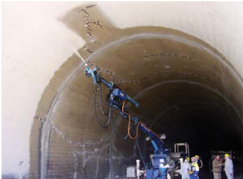
Fig. 4: Application near tunnel portal, Chekka Tunnel
