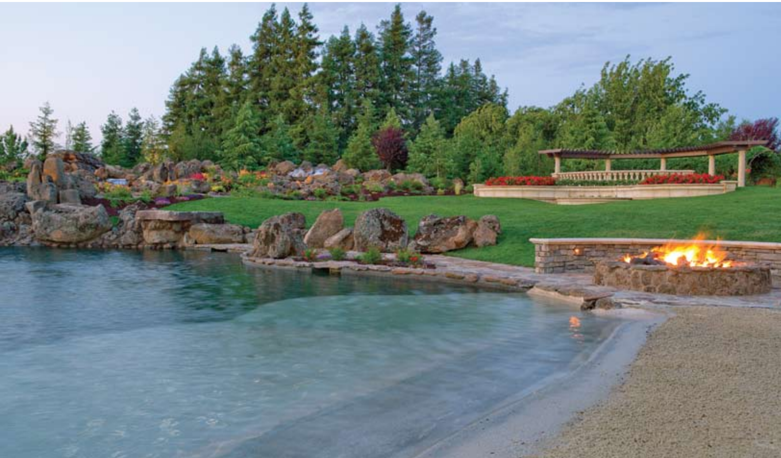
Fig. 3: Various colors of river rock exposed aggregate were used in the plaster for the pool to create a visual transition between the shallow and deep ends of the pool
