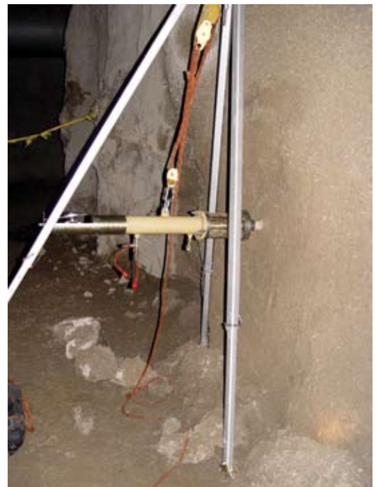
Fig. 8: Hydraulic jacking arrangement
