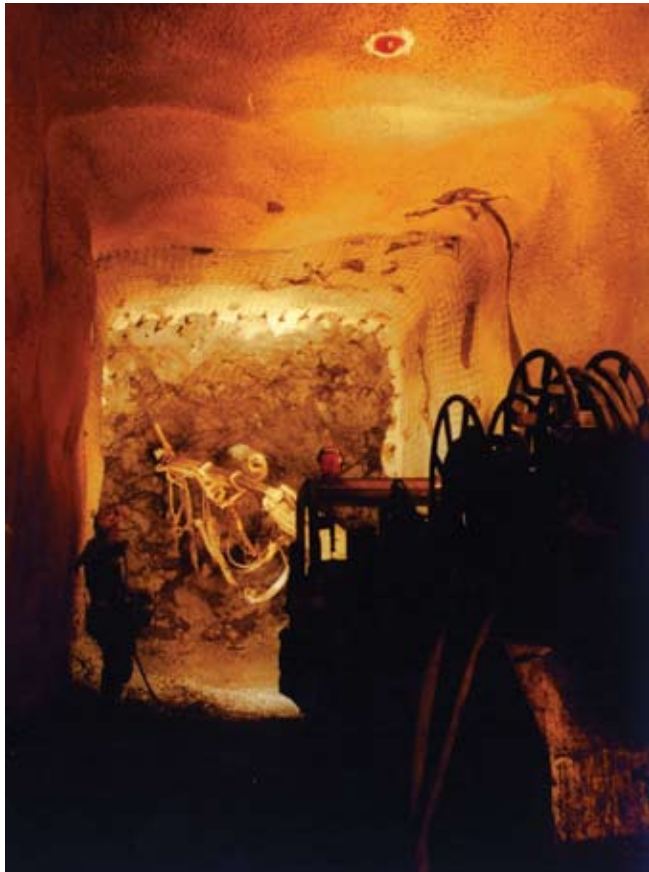
Fig. 1: Remote in-cycle shotcrete application
