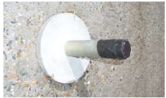
Fig. 4: Pull-out disc mounted ready to receive shotcrete
