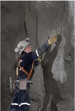
Fig. 4: Trowelling of finish shotcrete layer
