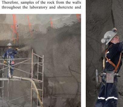
Fig. 3: Shotcreting of drift walls in progress
