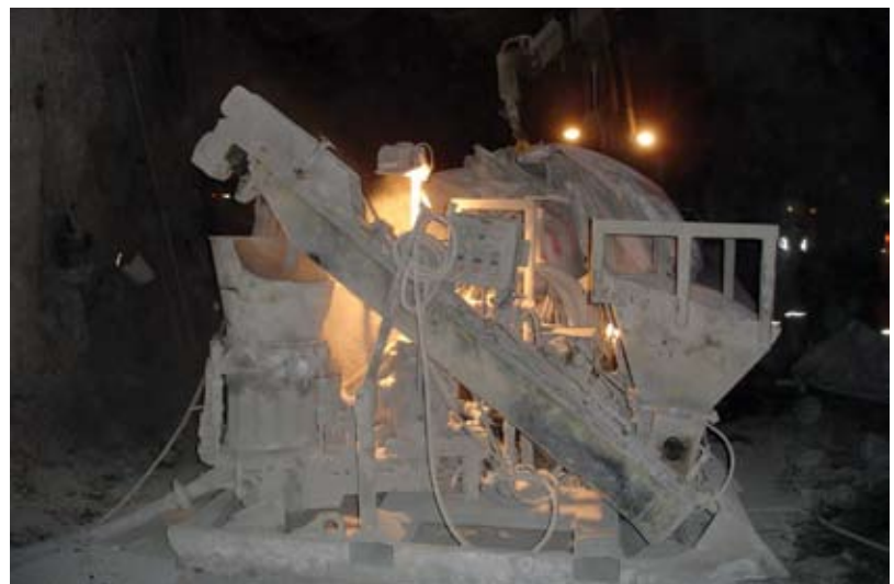
Fig. 3: Shotcrete predampener and gun
