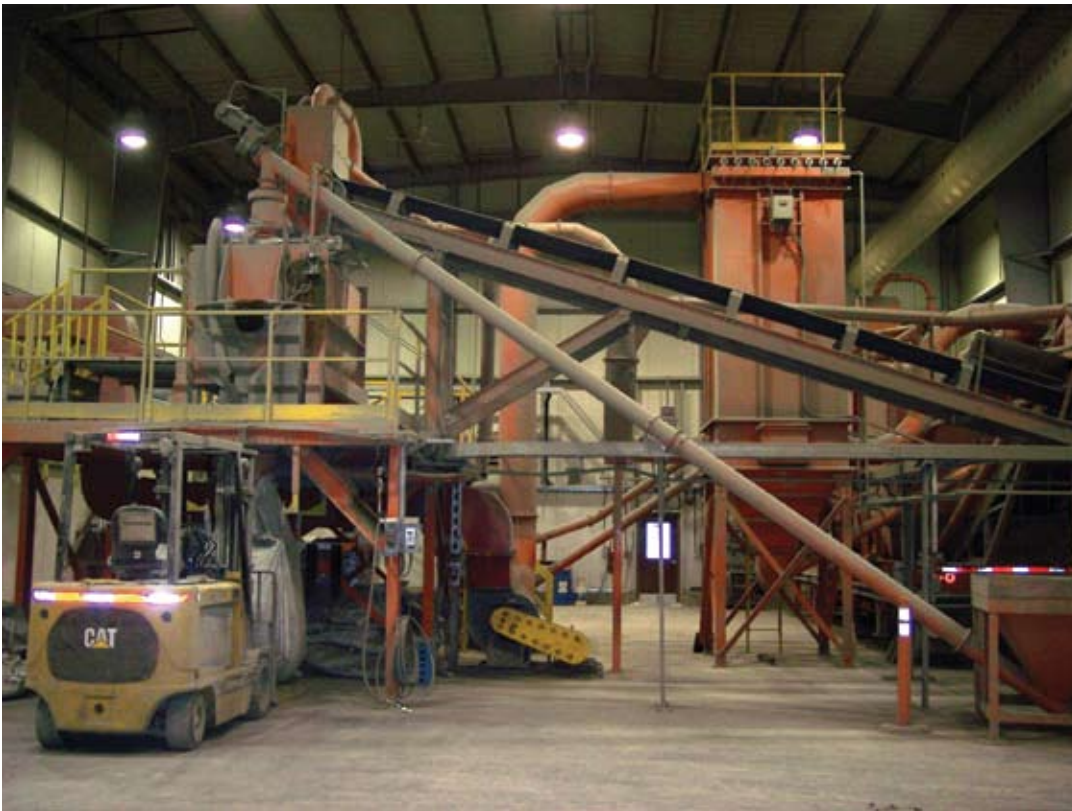
Fig. 2: Shotcrete manufacturing plant uses local aggregates and a concentrate shipped in over the ice road
