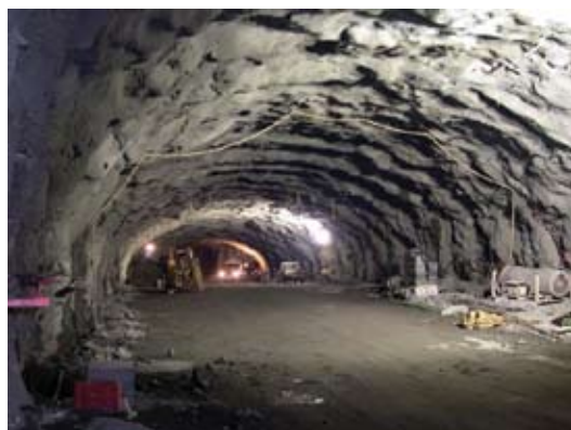
Fig. 2: Initial ground support shotcrete
