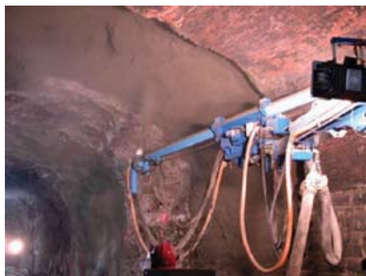
Fig. 1: Application of initial ground support shotcrete
