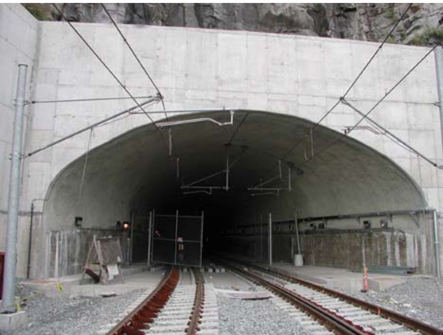
Fig. 9: Completed portal structure
