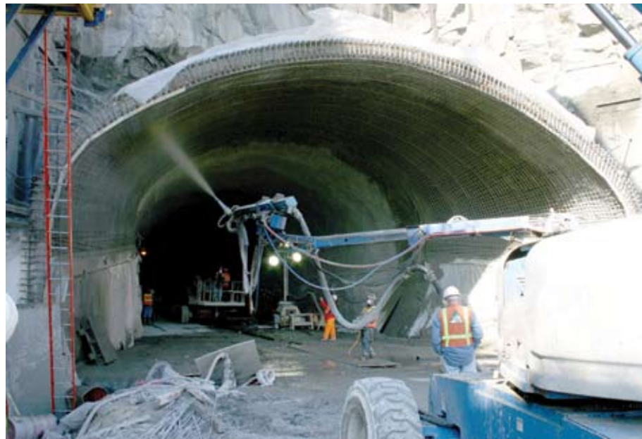
Fig. 3: Portal structure shotcrete application
