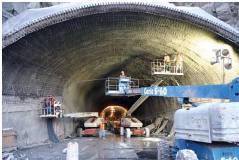
Fig. 4: Installation of second layer reinforcement
