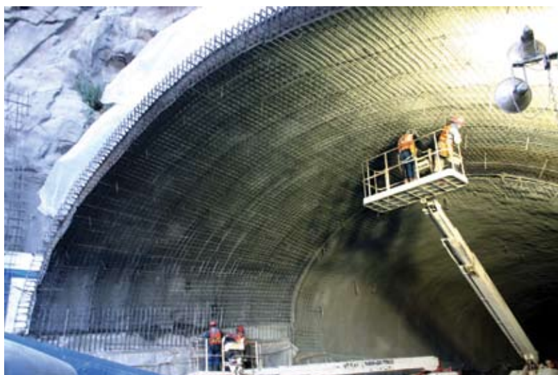
Fig. 7: Installation of second layer reinforcement in the open cut section
