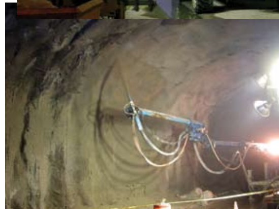
Fig. 8: Shotcrete application
