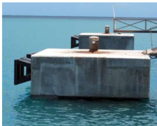
Fig.6: Concrete dolphins after shotcrete was placed and finished
