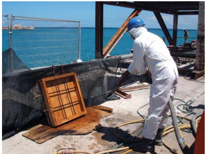
Fig. 2: Nozzelman preparing to shoot on-site test panels
