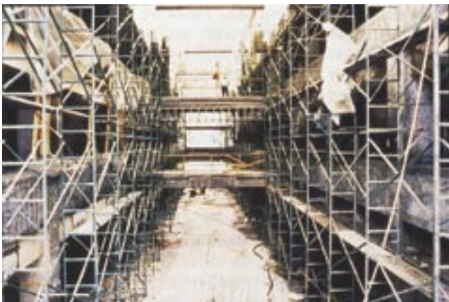
Interior atrium during construction
