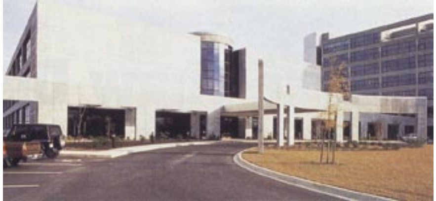
Completed Santee Cooper headquarters annex
