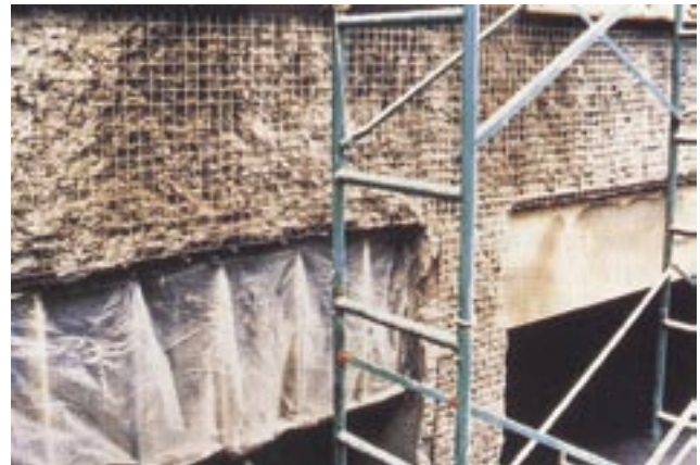
Surface area prepared for shotcrete placement
