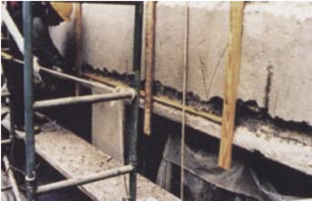
Interior forms for reveals
