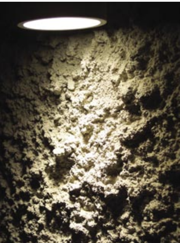
White cement shotcrete with a standard finish was carefully selected
