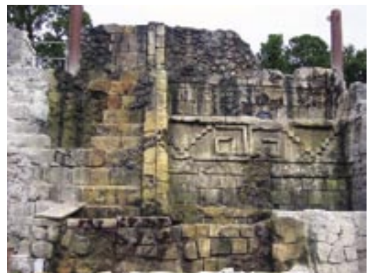
Coloration of the Mayan temple in Jacksonville progresses by using multiple layers of acrylic latex paint
