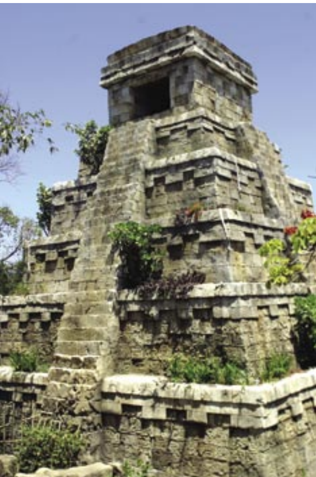
A shotcrete pyramid with authentic historical Mayan detail
