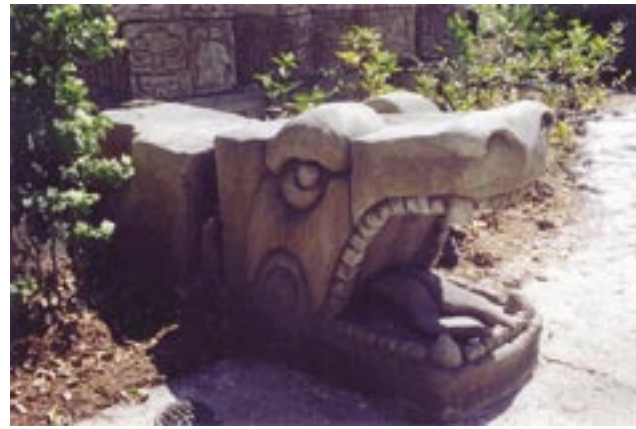
A sculpted Mayan dragon head ornament formed in shotcrete and reinforcing bar
