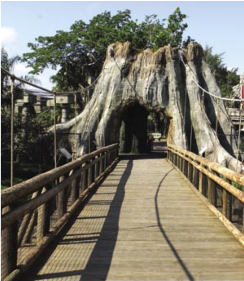
A shotcrete jungle ficus tree serves as the entrance to Dreyer Park Zoo's Tropics of the Americas exhibit
