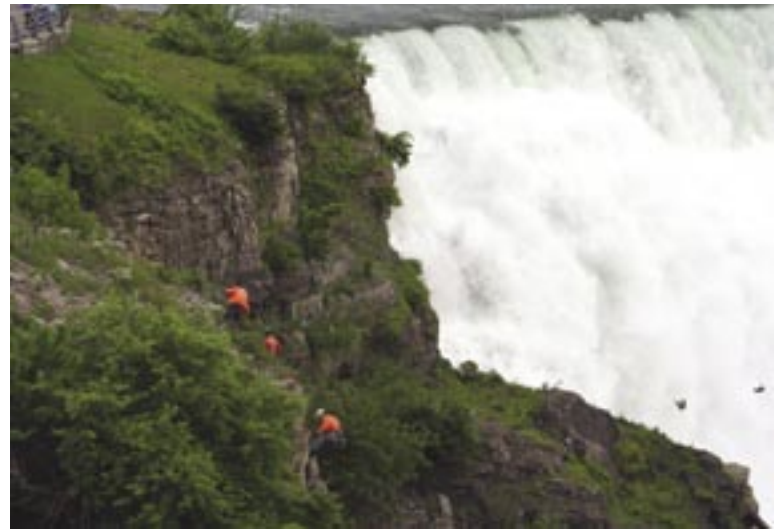
Crew scaling rock from the slope
