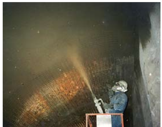
Fig. 6: Acme 2 in. (50 mm) nozzle/Staten Island Terminal Tunnel (Photo courtesy of George Yogy)
