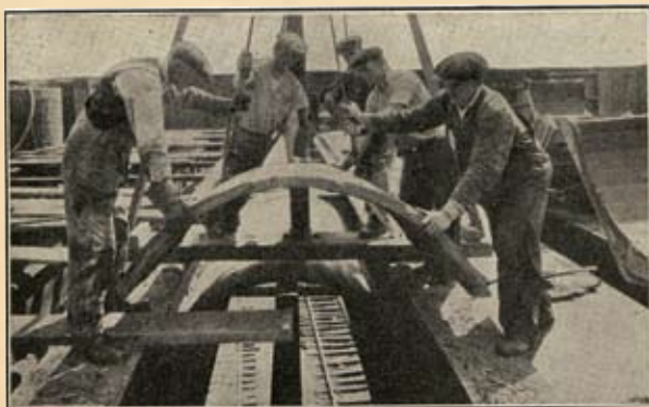
FIG. 5—SETTING PRE-SHOT GUNITE ARCH SLAB ON P.R.R. BRIDGE
