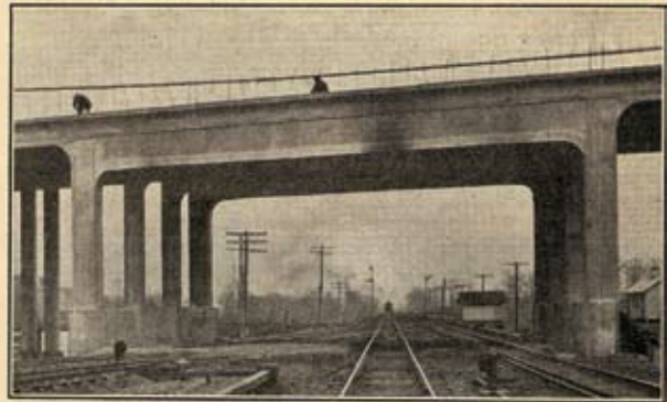
FIG. 2—AULON VIADUCT, MEMPHIS, TENN.
