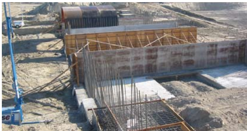
Stemwall and arch forms
