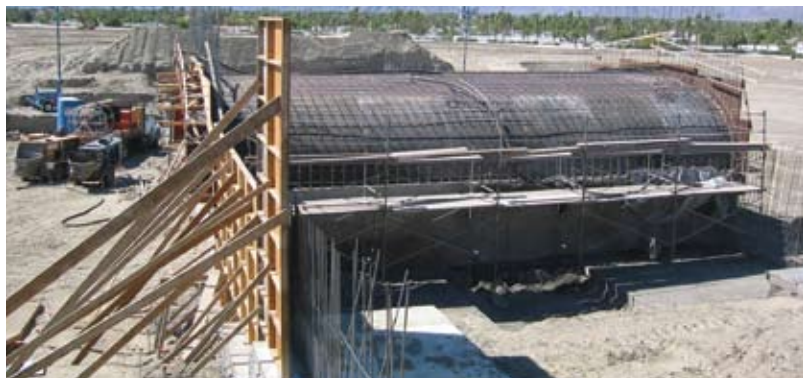
Arch ready for shotcrete
