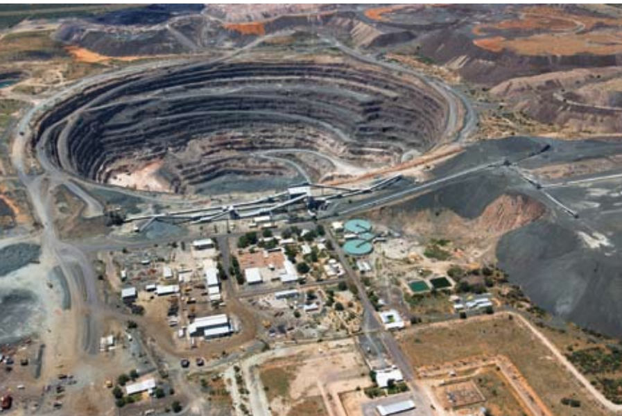
Process Plant of Debswana
