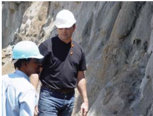
Evaluation of shotcrete application
