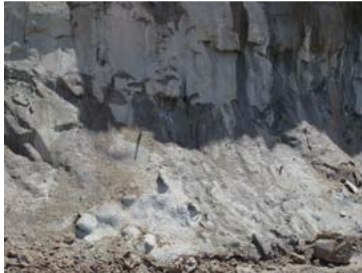
First shotcrete trials
