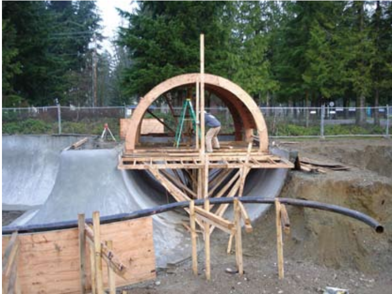
Construction of fullpipe
