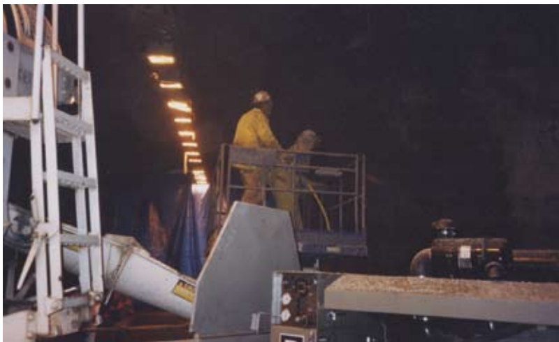
Fig. 1: Colorado Dept of Transportation Highway 6, Denver, CO
