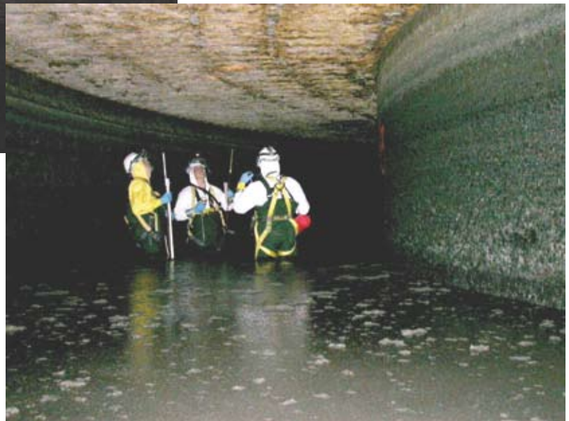
Fig. 7: Box tunnel roof repair
