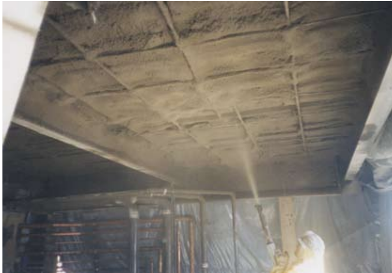
Fig. 6: Hospital roof, Pueblo, CO
