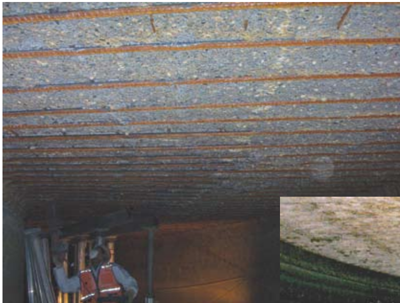
Box tunnel roof repair
