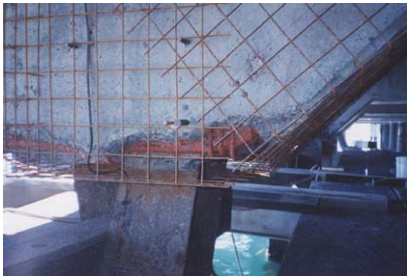
Fig. 5: Container ship pier project, Kodiak, AK
