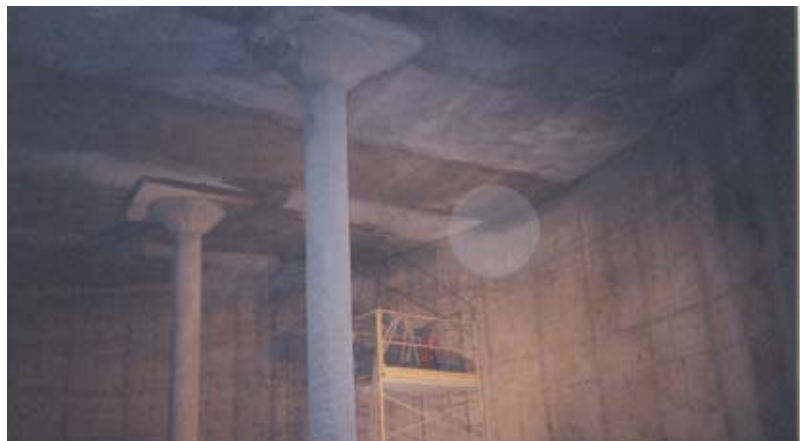
Fig. 2: Roof of water tank, Vail, CO
