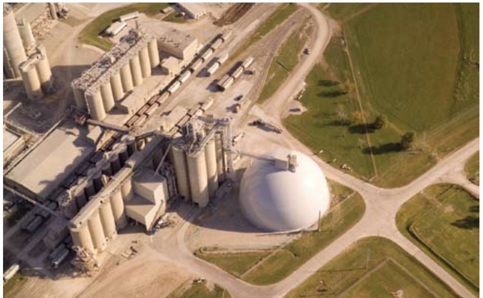
Fig. 2: Ashgrove Cement Facility, Chanute, KS
