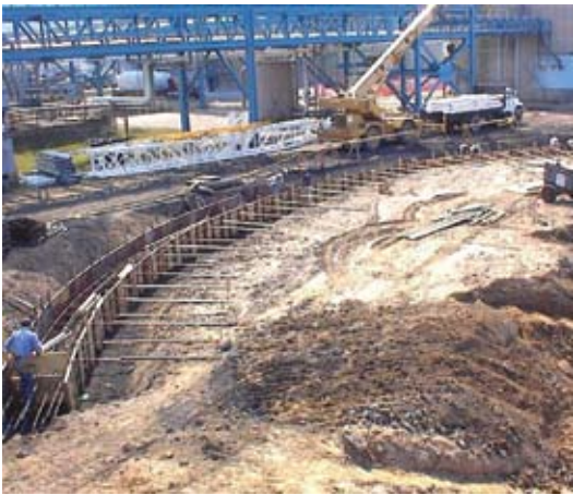
Fig. 3: Construction of ringbeam footing
