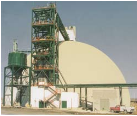
Fig. 9: Holcim Cement Plant, Clarksville, MO
