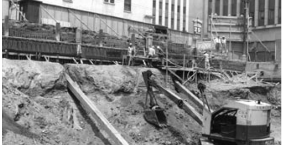
Gunite shoring and basement wall project using dry-mix shotcrete, 1955
