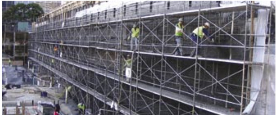
Gunite shoring and basement wall project using wet-mix shotcrete, 2005
