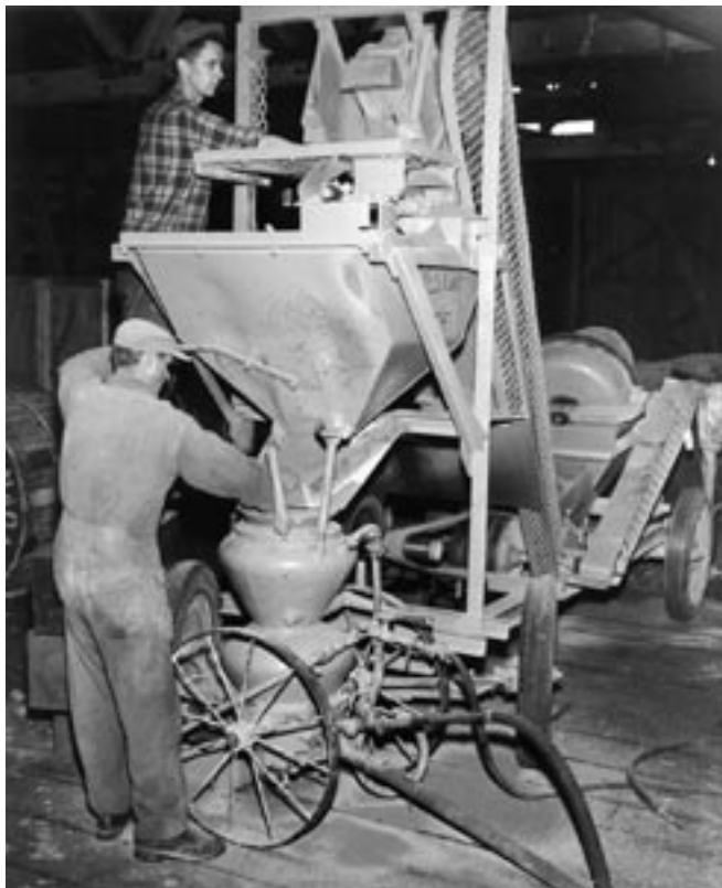
Double chamber dry-process shotcrete machine used on seismic retrofit project, 1954
