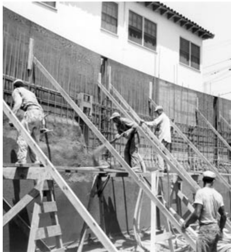
Structural retaining wall project using dry-mix shotcrete, 1955
