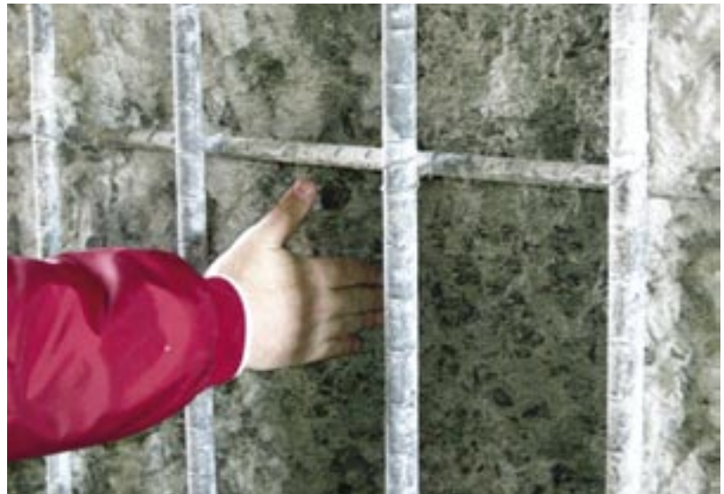
Deep repair after removal of unsound concrete
