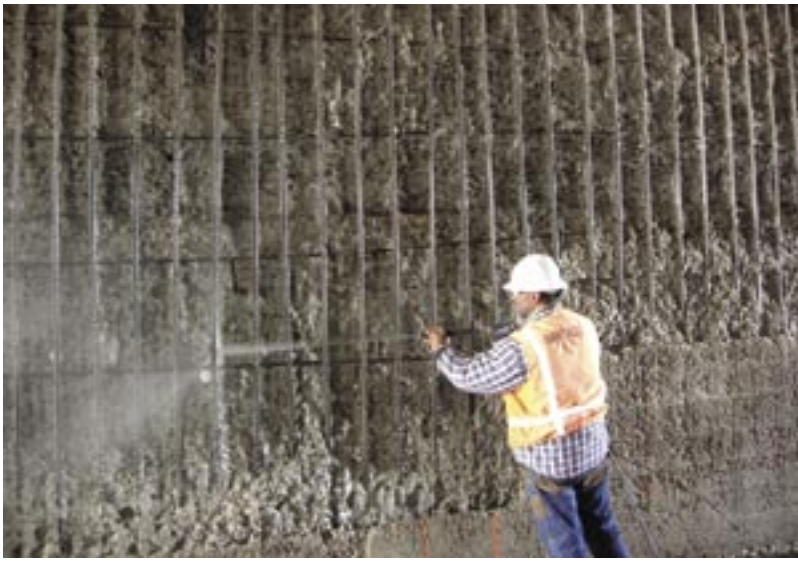
Final surface preparation
