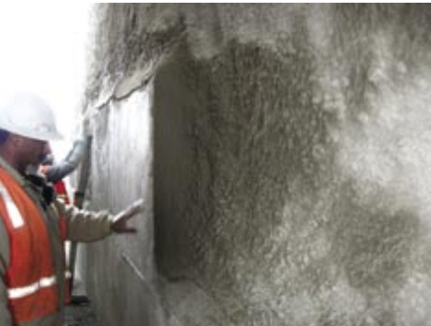
Final finishing of the shotcrete repair. Note the 8 in. depth
