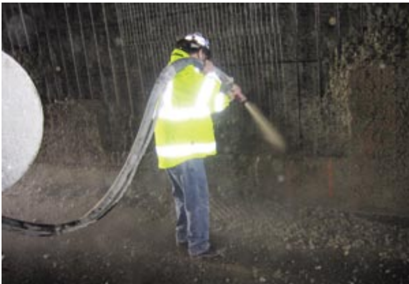
Installation of shotcrete over welded wire mesh at test section
