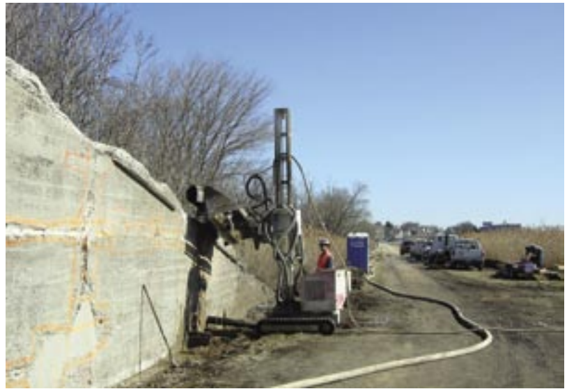
Hydrodemolition robot preparing to remove unsound concrete
