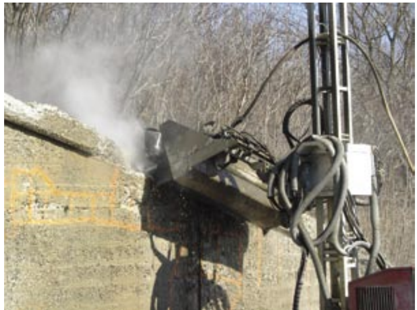
Hydrodemolition robot removing unsound concrete
