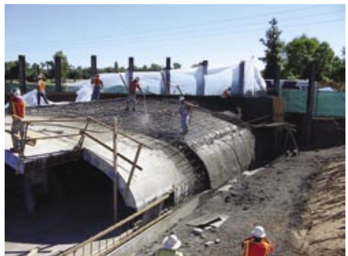
Placing shotcrete on Con-Arch steel forms
