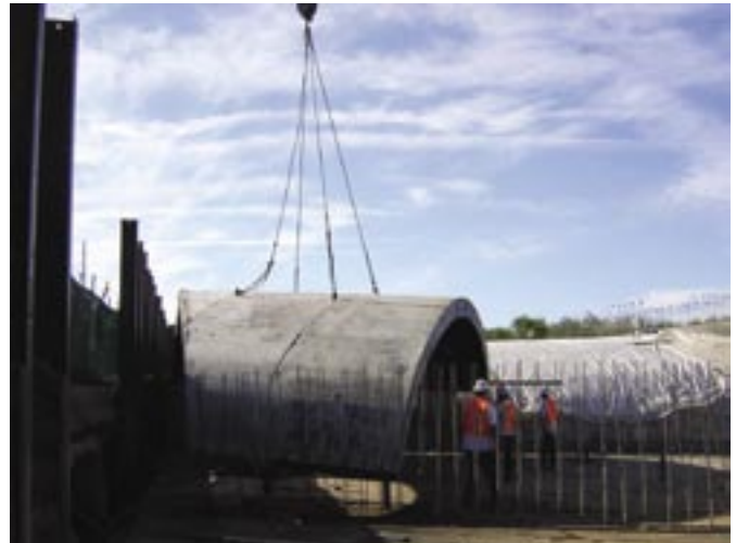
Setting skewed 42 ft Con-Arch steel form
