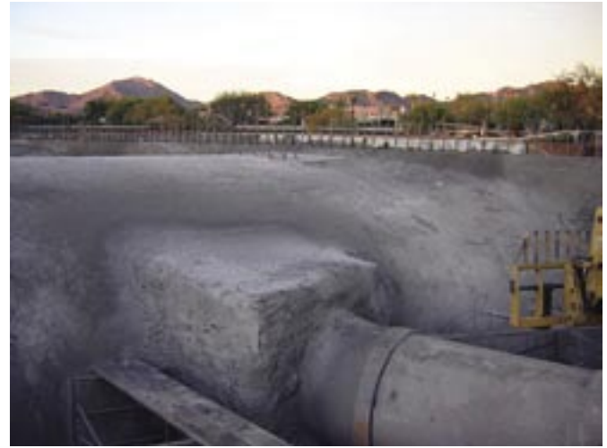
Shotcrete collar pipe penetration
