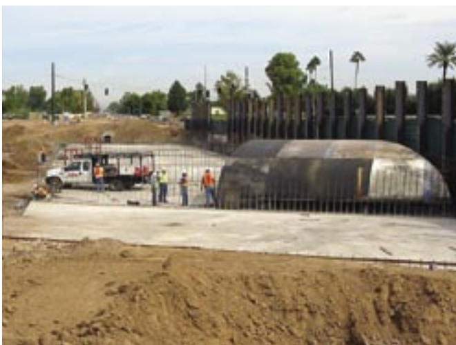
Setting Con-Arch reusable steel forms
