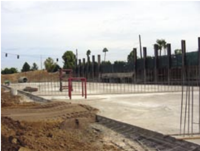
Concrete invert poured ready for form placement
