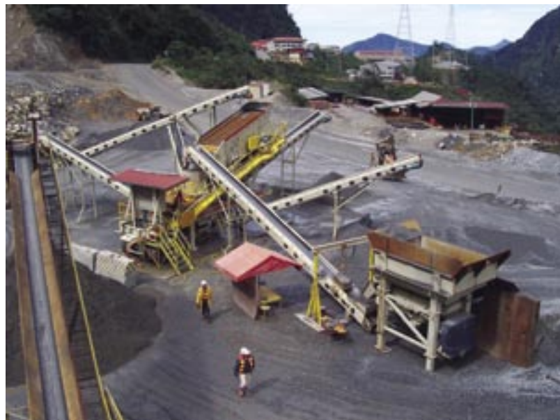
An overview of PT Freeport's NW7100 at Milepost 72
