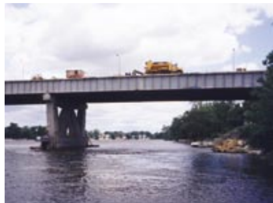
Fig. 3: Dry-mix shotcrete supplied with concrete mobile mixer for pier repairs of bridge over Rivière-des-Prairies River, Montréal, QC
