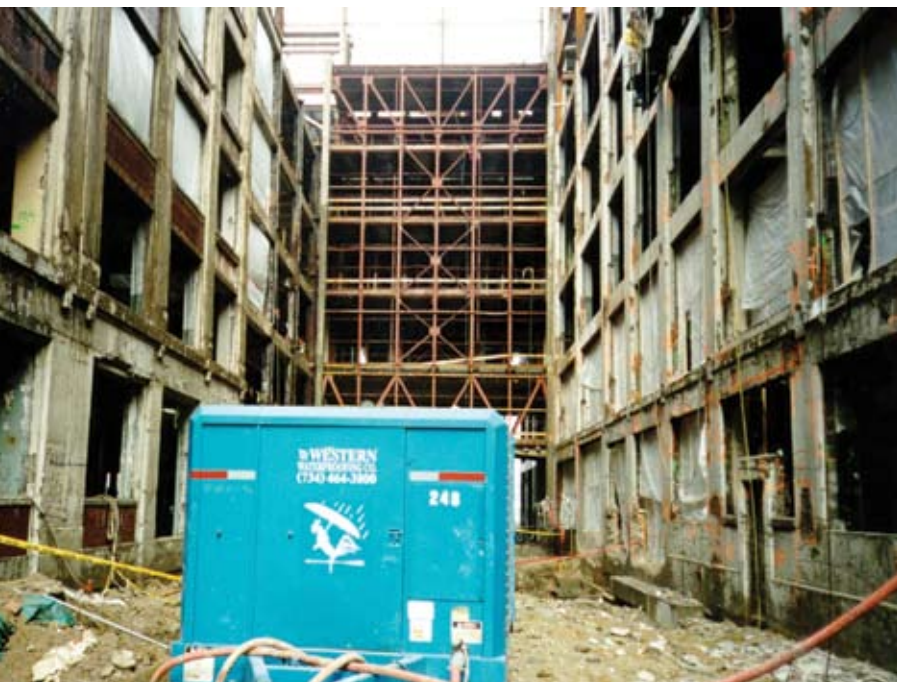
Condition of the two 1920s-era buildings
