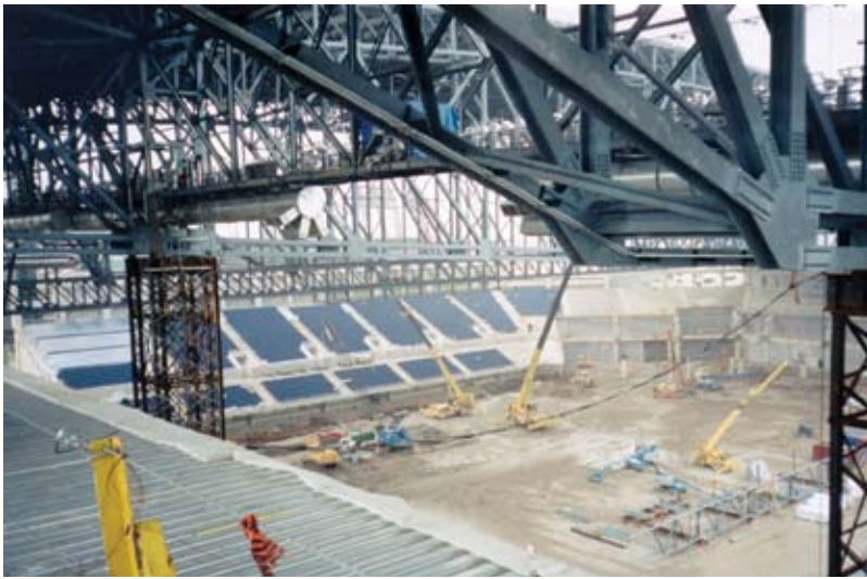
Inside view of Ford Field during construction
