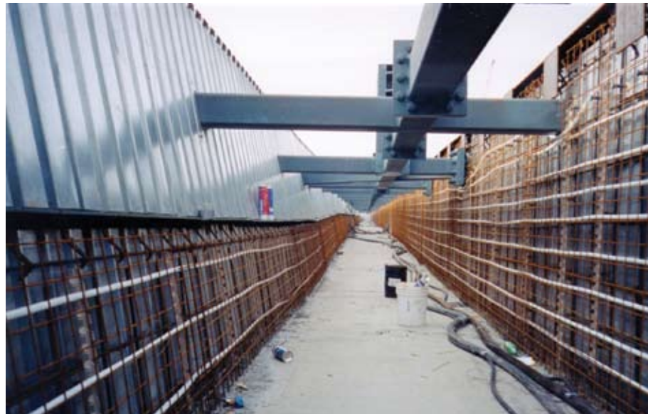
Inside view of southern elevation roof trough prior to shooting
