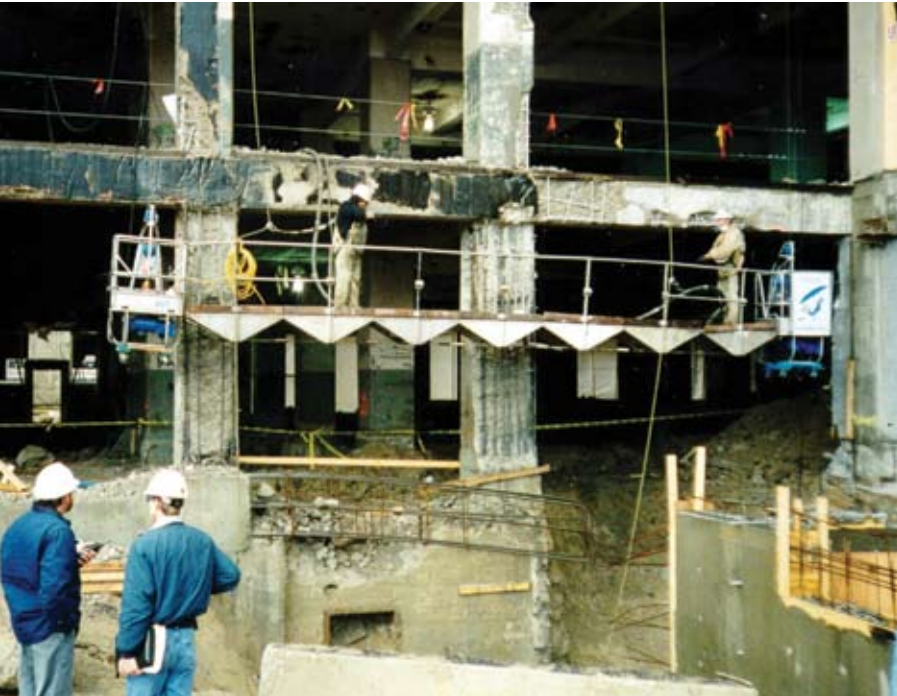
Early work on the old Hudson warehouse
