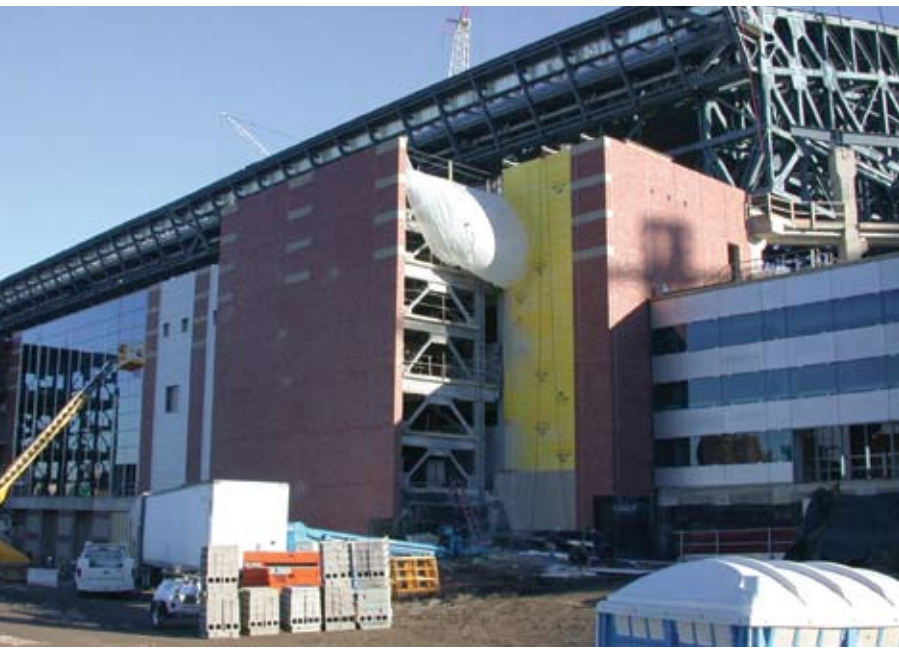
Overview of north elevation showing the roof trough
