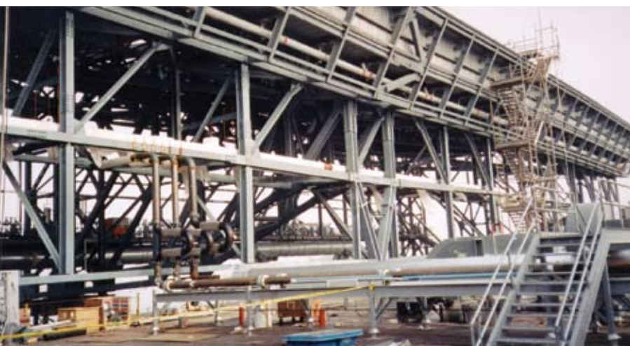
South elevation roof trough, prior to shooting
