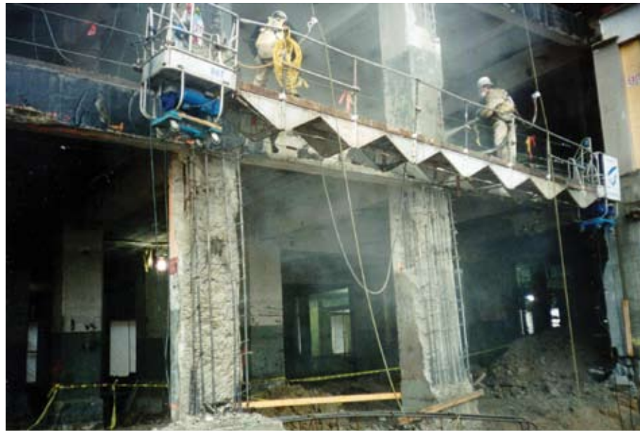
Shotcreting the columns of the old structure
