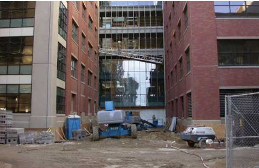
Further progress of the Hudson warehouse buildings
