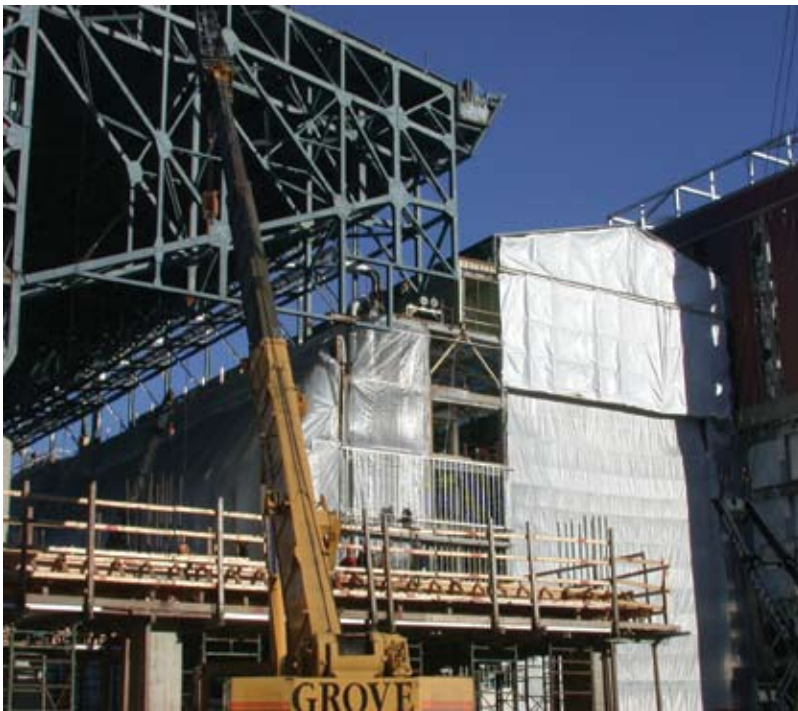
Southern trough above the old warehouse section
