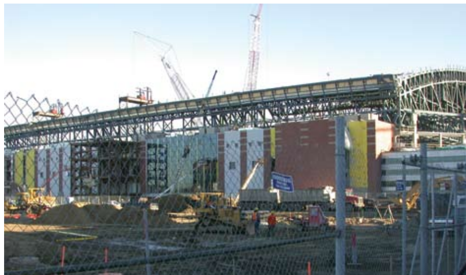
Overview of north elevation showing the roof trough
