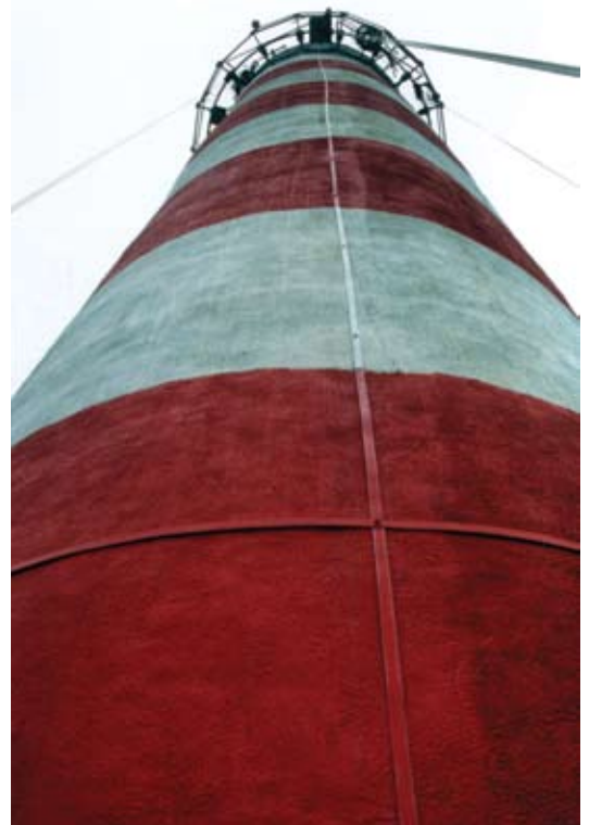
Repaired refinery chimney shaft (500 ft [150 m] high)
