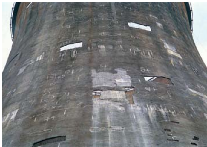
Replacement of concrete in the so-called "damaged windows" of cooling towers
