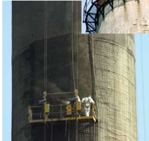
Middle zone of the chimney during shotcrete application on meshed base
