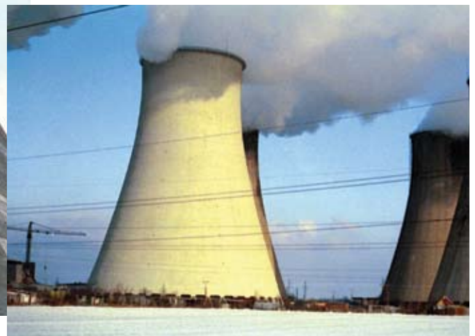
Cooling tower after repair
