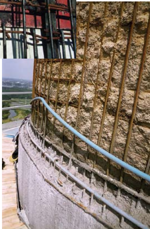
Completion of finish casing on double reinforcement
