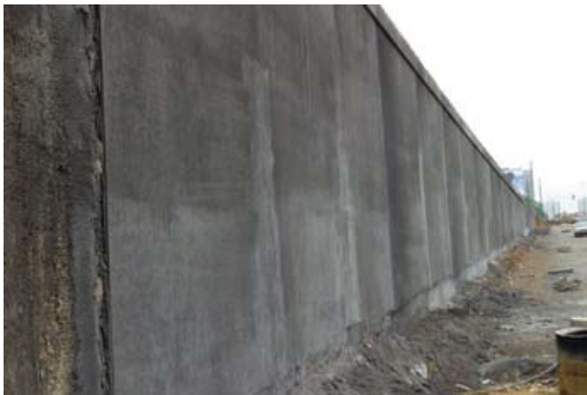
Shotcrete on tunnel diaphragm walls
