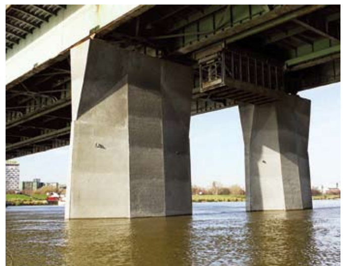
Supports after a repair with shotcrete
