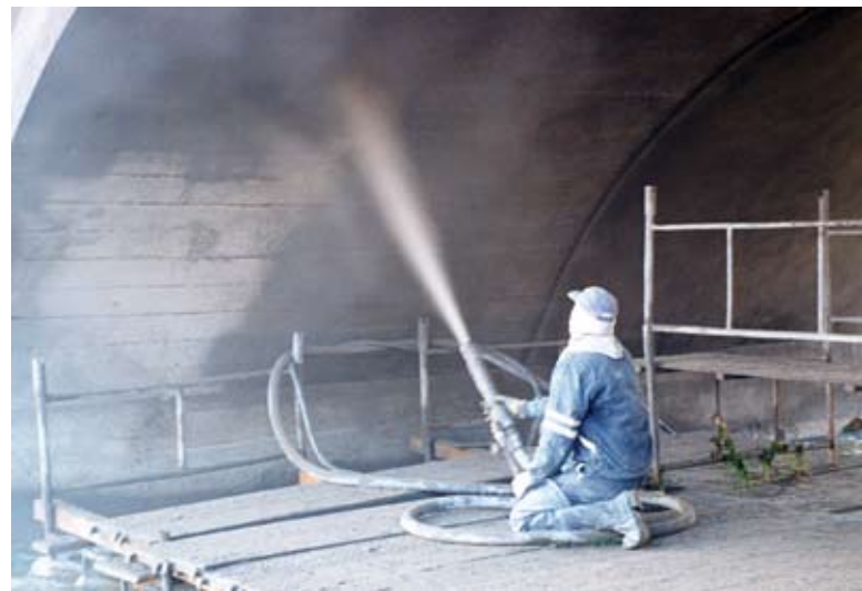
Repair of arch bridge vault
