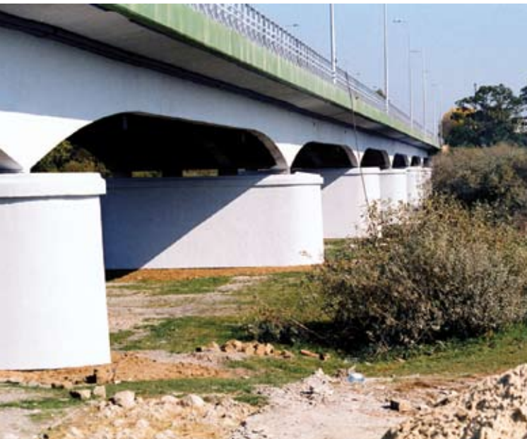
Complex repair of a bridge
