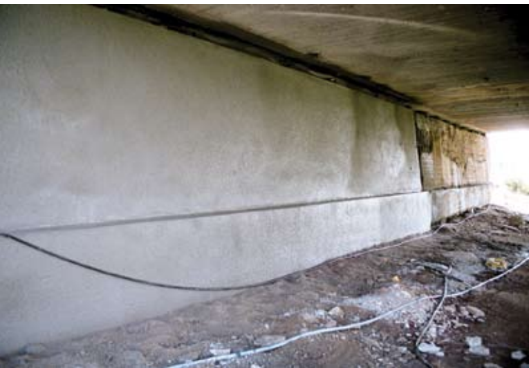
Abutment before and after repair
