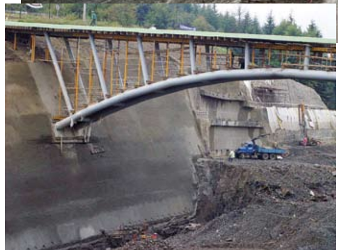
Strengthening of excavation slope on the border of Slovakia
