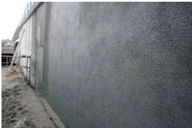
Shotcrete on a retaining wall
