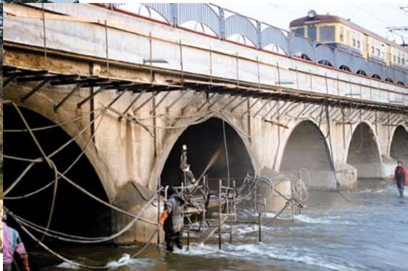
Repair of historic bridge
