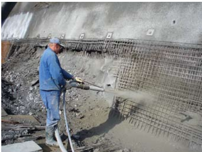
Slope strengthening in deep excavation
