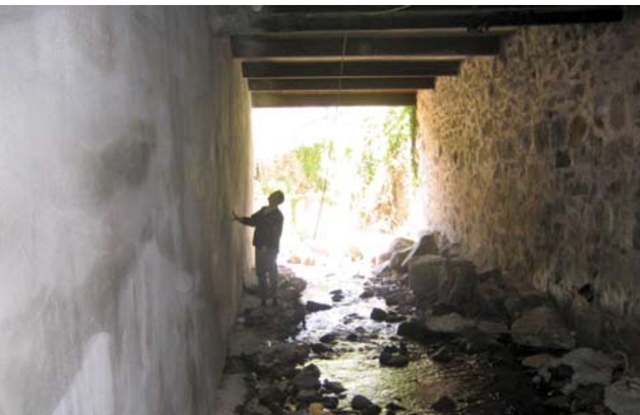
Operations Manager Timothy Hill, PE, inspects the tunnel
