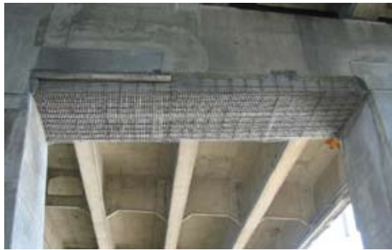
Fig. 6: Mesh installation—Île-aux-Tourtes Bridge
