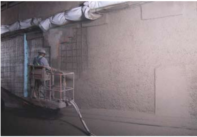
Fig. 9: Curing system already in place while shotcreting
