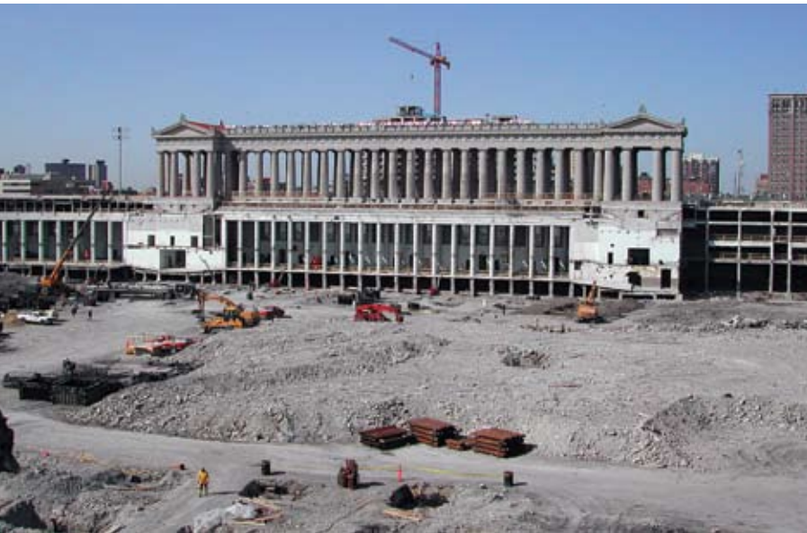
View of the stripped structure from the east
