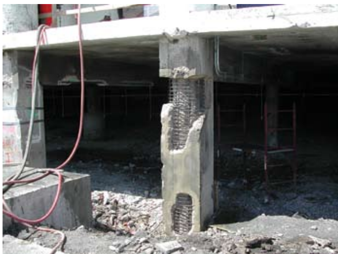
Original mock-up preparation
