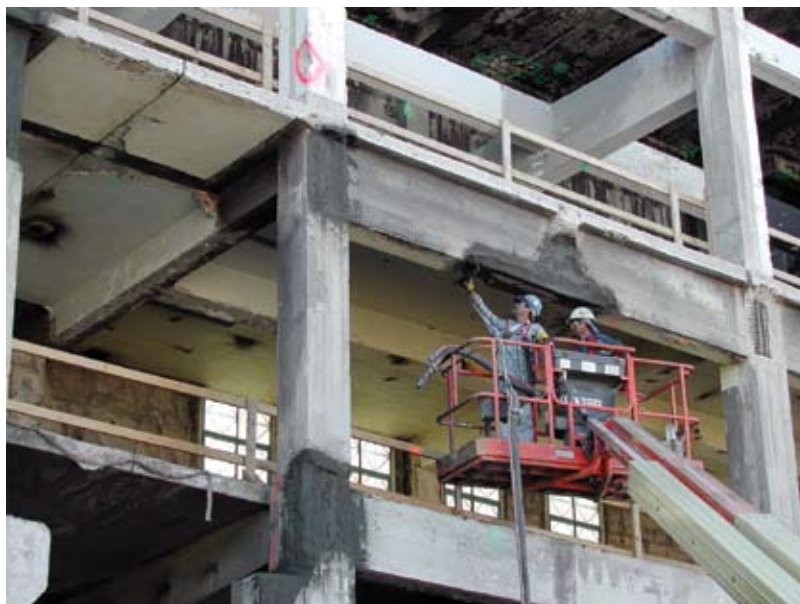
Finishing shotcrete on mezzanine underside
