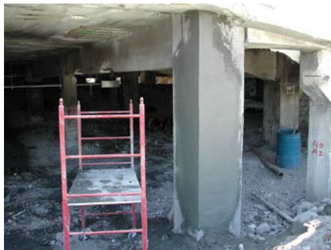
Finished column mock-up
