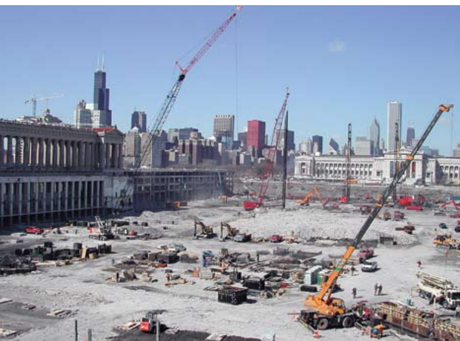
Looking north—demolition complete on the west side
