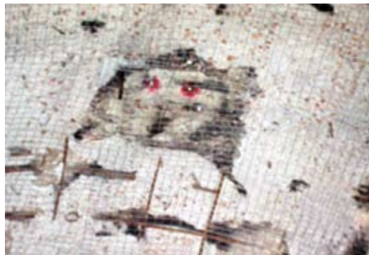
Typical spalled area for repair with welded wire installed
