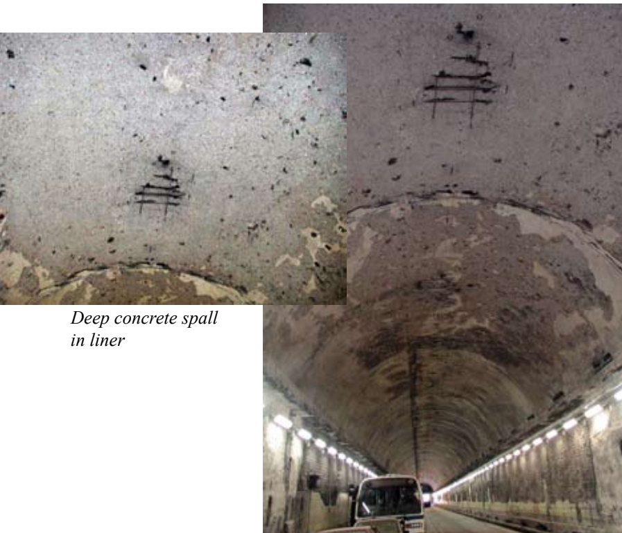
Typical structural damage from fire tests
