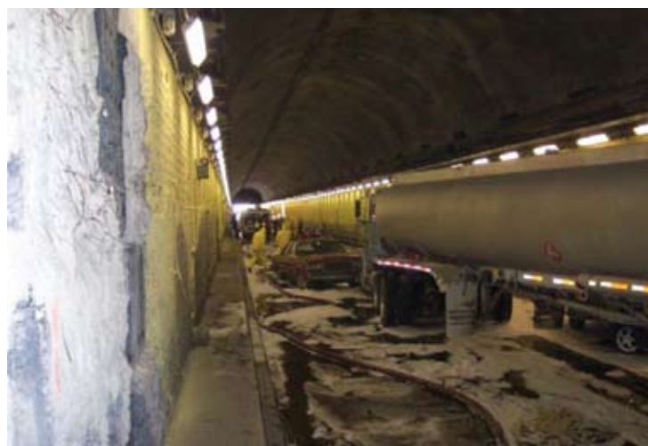
Highway incident training area
