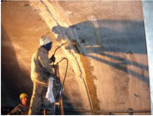
Typical chemical grout injection for tunnel joints
