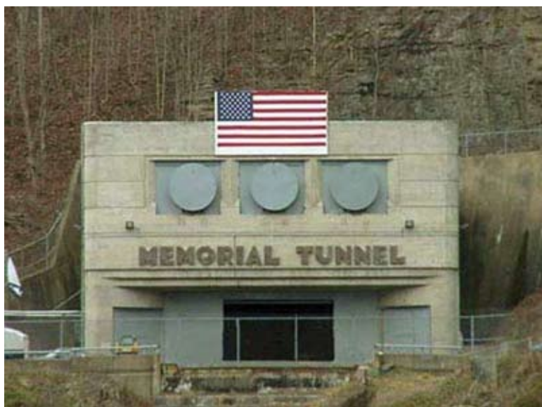
East portal of the Center for National Response (Memorial Tunnel)
