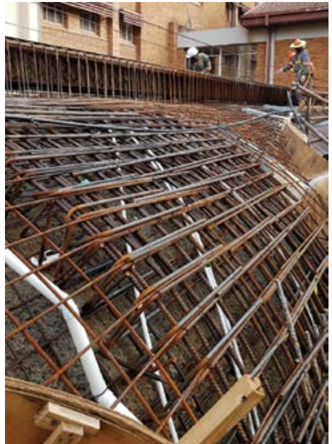
Fig. 3: Complex reinforcing steel for the canopy
