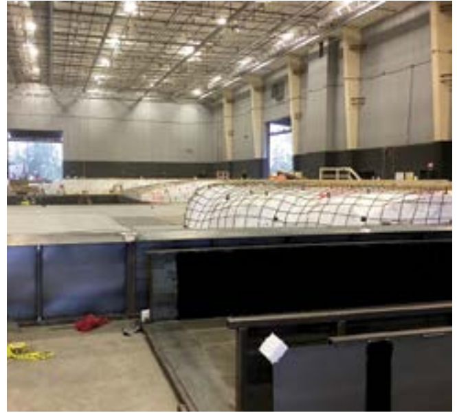
Fig. 3: Stainless steel cofferdam around set
