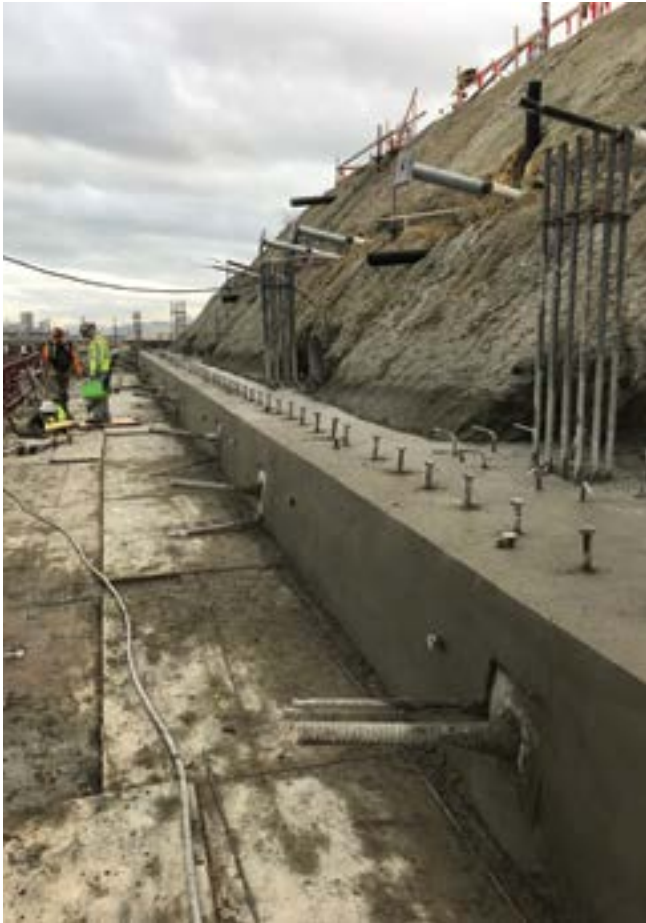
Fig. 3: Finishes on grade beam
