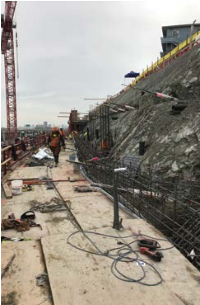
Fig. 1: Grade beam with work platform
