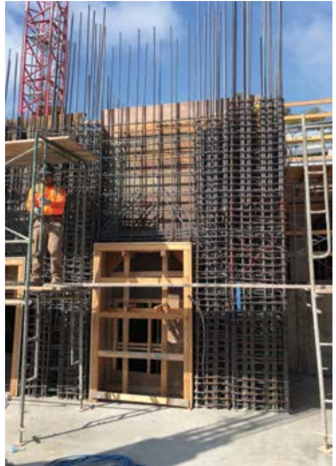
Fig. 4: Typical shear wall and boundary elements
