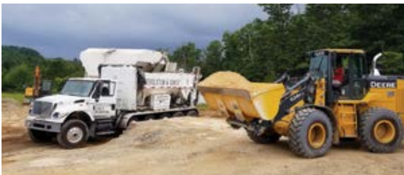
Fig. 1: Local aggregate staging area for volumetric batch trucks
