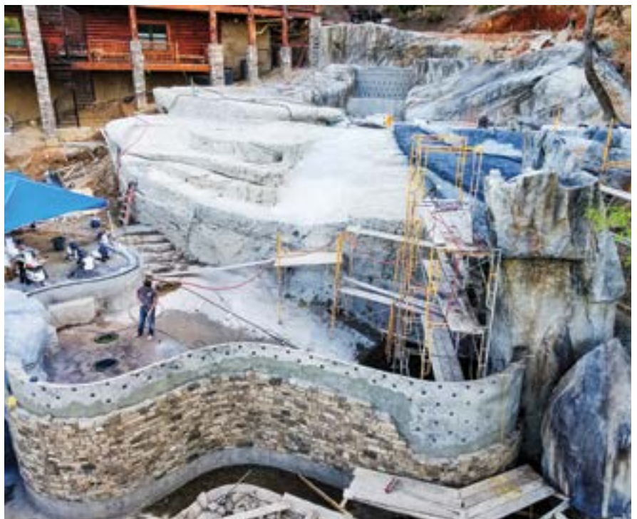
Fig. 5: Overview of the project near completion
