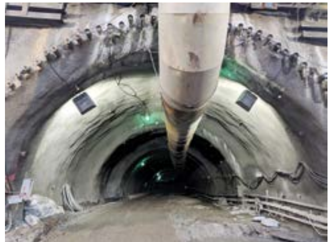
Fig. 2: Plymouth Tunnel East Portal top heading excavation
