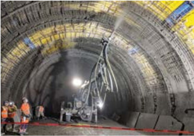
Fig. 5: Spraying secondary liner overhead arches on PVC waterproofing membrane
