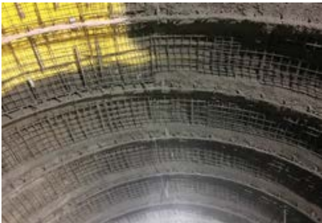
Fig. 6: Secondary liner overhead arches built up on lattice girders
