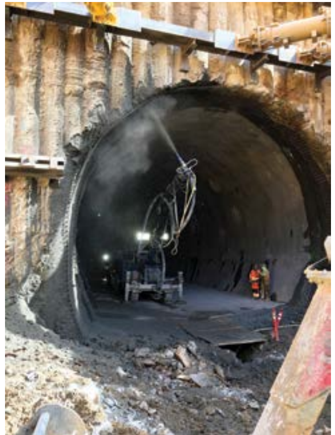
Fig. 4: Completion of initial lining after excavation
