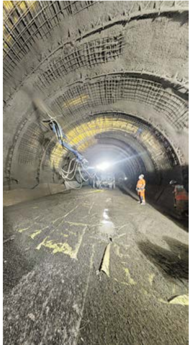
Fig. 7: Spraying secondary liner bays between arches
