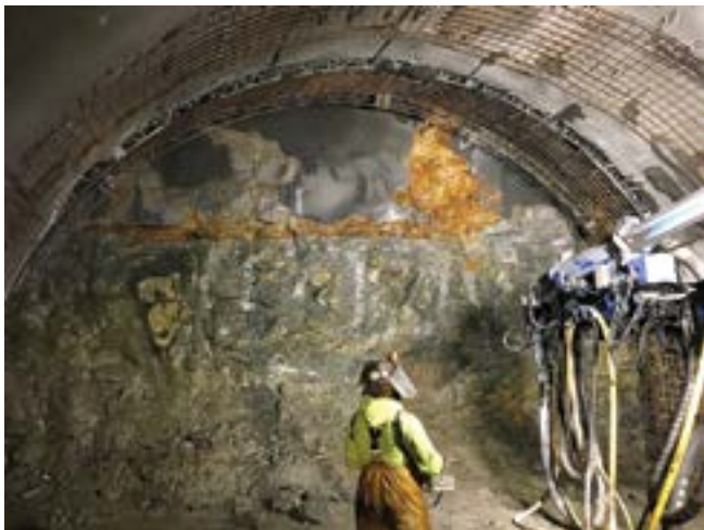
Fig. 3: Top heading flash coat application in mixed face conditions
