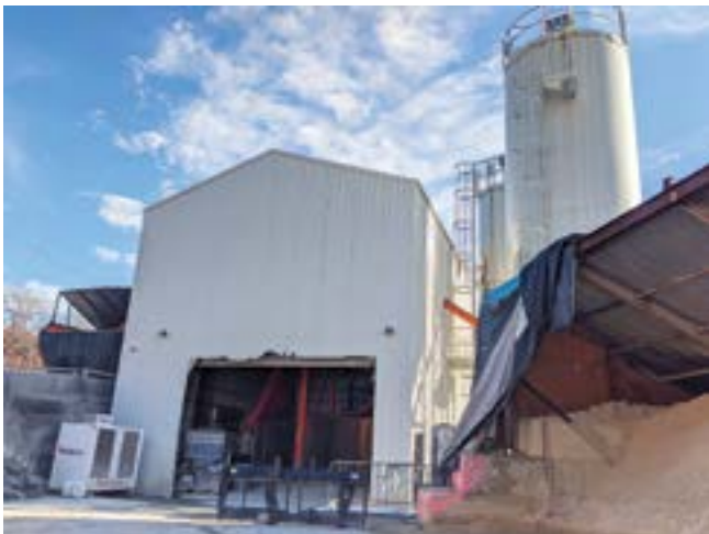
Fig. 1: ACT WiCoMix WM 1500 Batch Plant with buildings and silos
