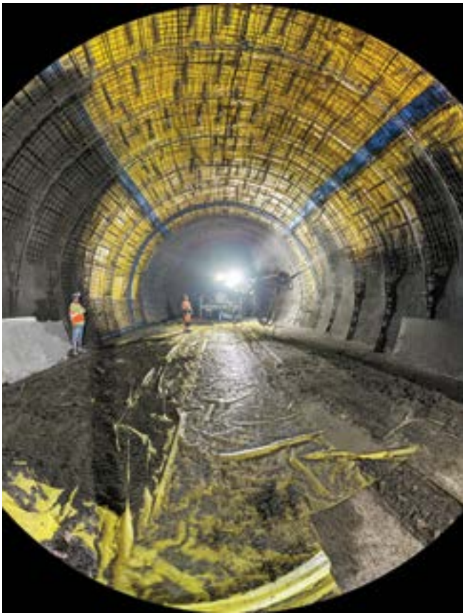
Fig. 9: Initial shotcrete application on PVC liner
