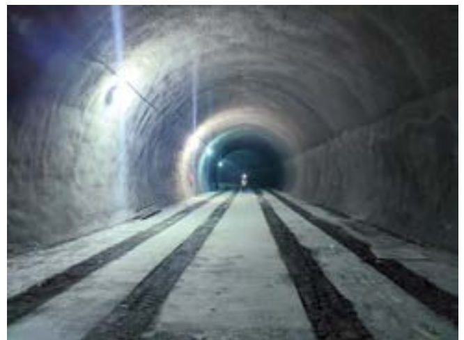
Fig. 8: Plymouth Tunnel shotcrete final liner with form-and-pour invert
