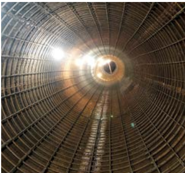
Fig. 4: Reinforcing bar installed
