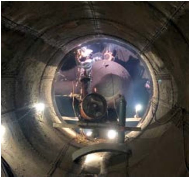
Fig. 3: Welding steel transitions at upstream and downstream shotcrete terminations
