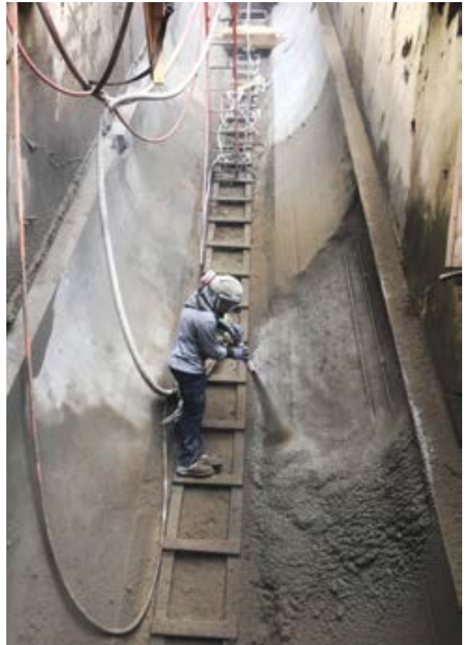
Fig. 4: Shooting side of basin off middle strip
