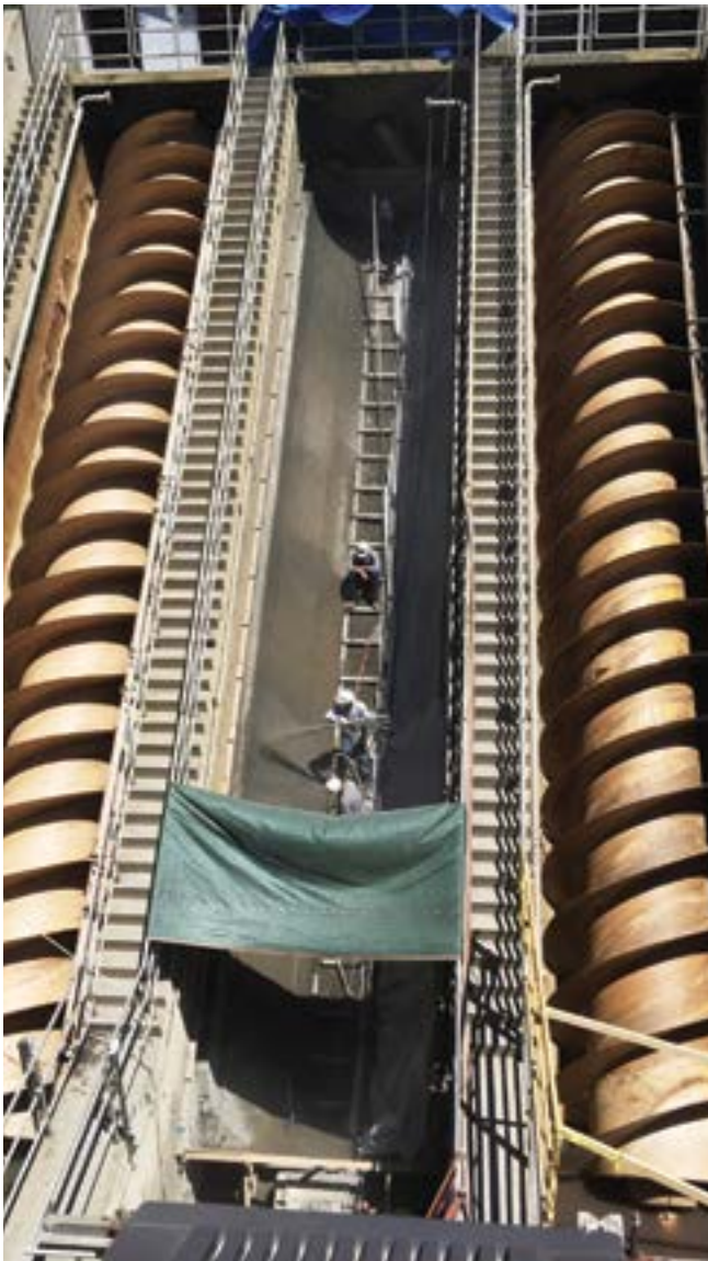
Fig. 5: Overview of shooting the basin with access down the middle
