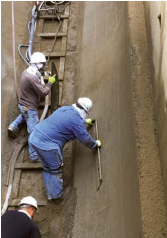
Fig. 3: Careful trimming of the sides
