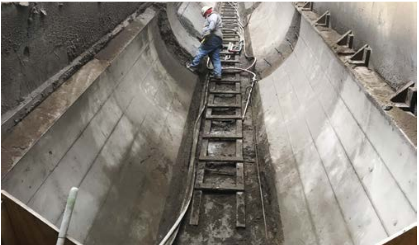
Fig. 2: Basin walls shot with guidewires in place
