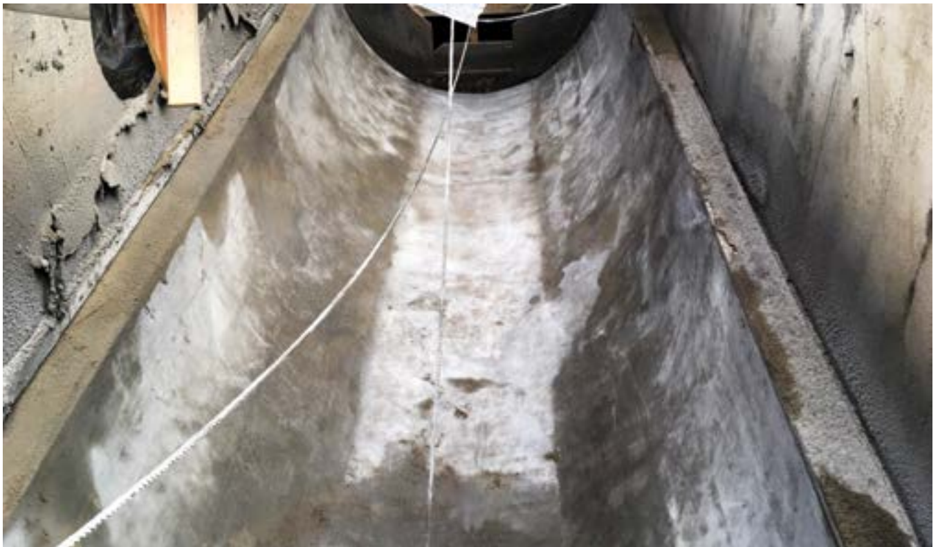
Fig. 1: Finished screw pump basin with tight radius
