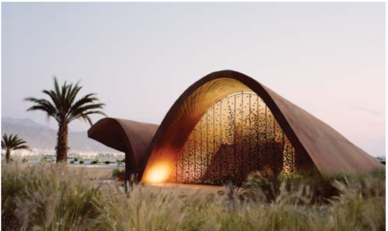
Fig. 4: The shotcrete was mixed with local materials and dyed with a pigment sourced from the nearby hills, further linking the building with the landscape (Photo courtesy of Rory Gardiner)
