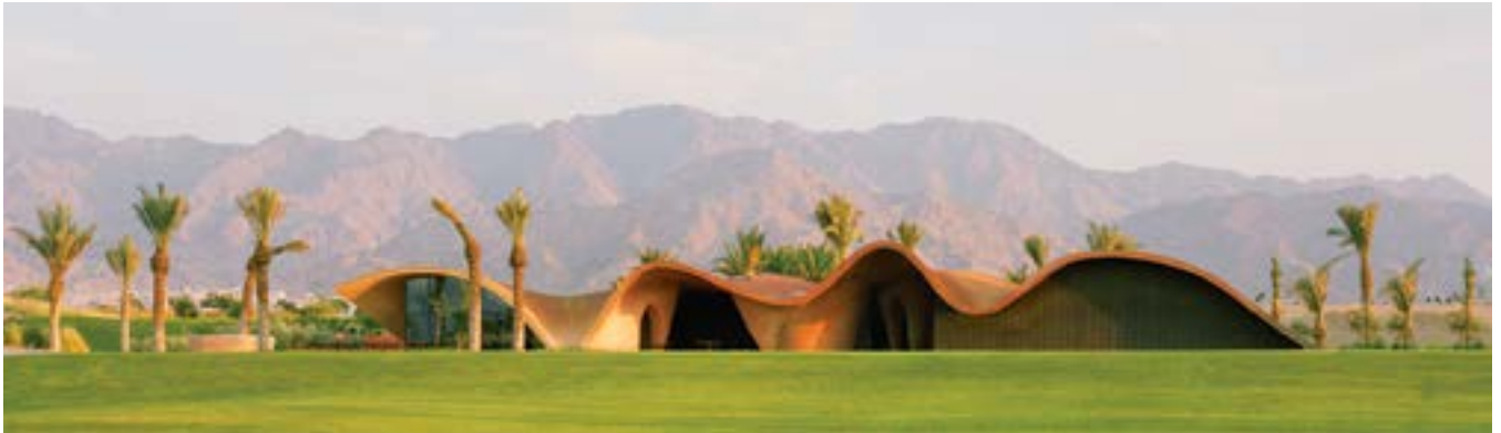
Fig. 1: The building's rolling, dune-like form evokes the beauty of the surrounding desert and mountains (Photo courtesy of Rory Gardiner)
