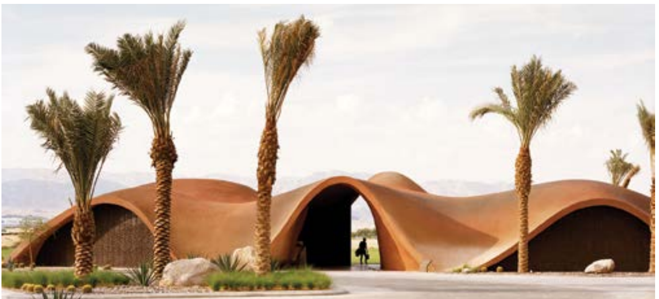
Fig. 2: A continuous shotcrete shell emerges from the sand, enveloping the volumes and defining the various program areas (Photo courtesy of Rory Gardiner)
