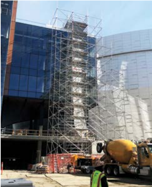
Fig. 3: Self-supporting scaffold tower
